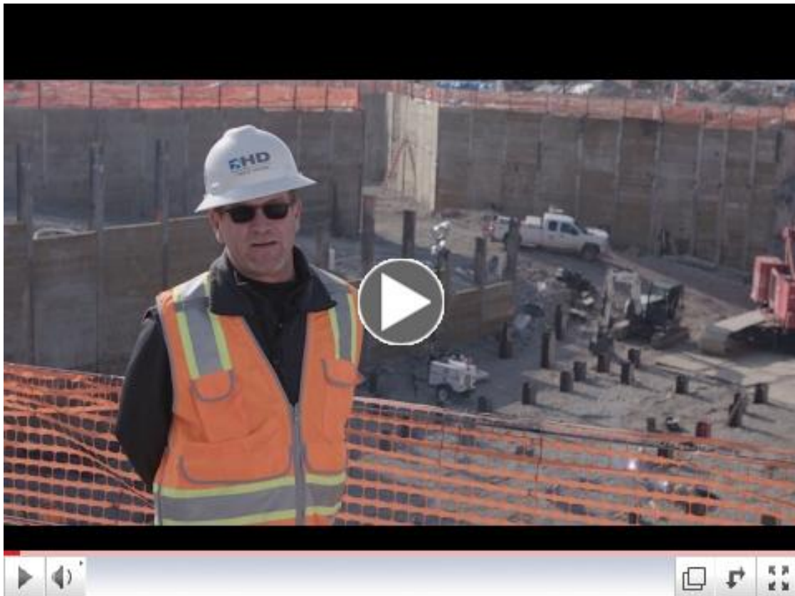
Steel Pile Installation
