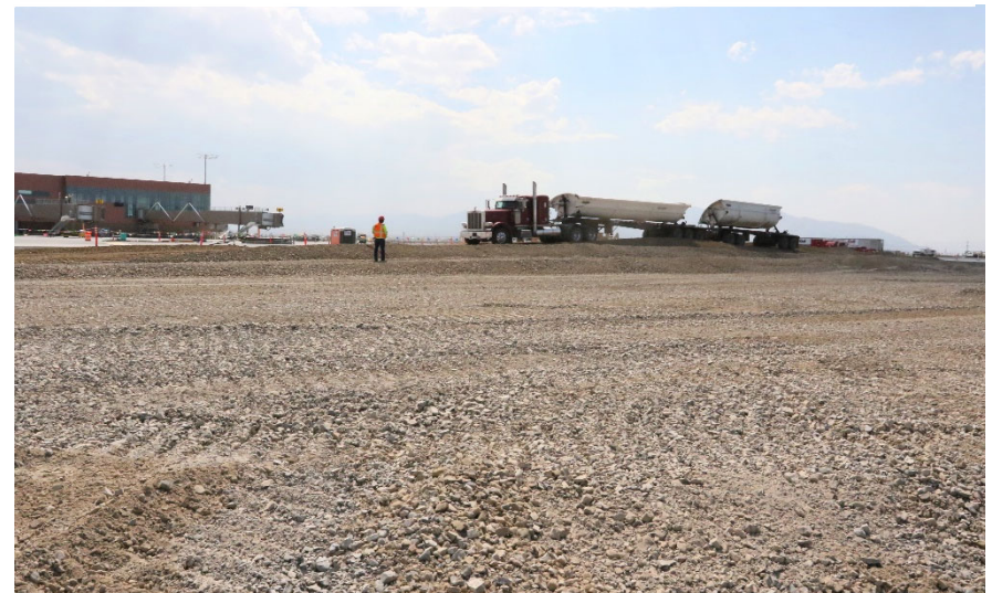
P4 Hardstand Sitework
