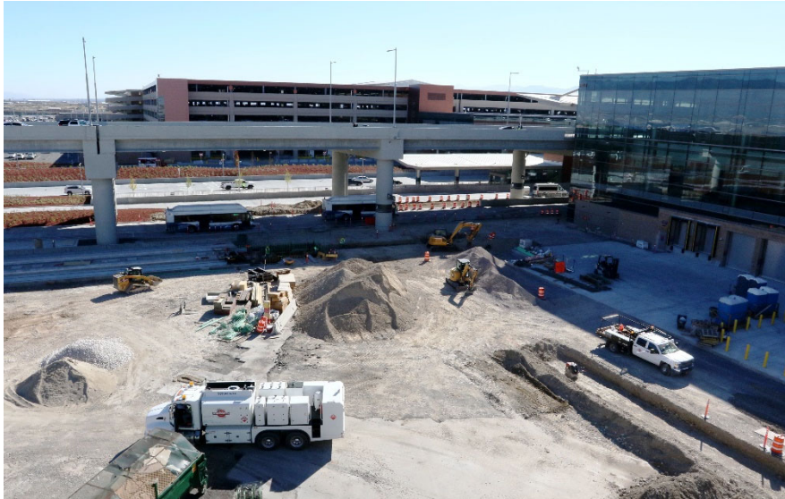
TRAX Platform Construction
