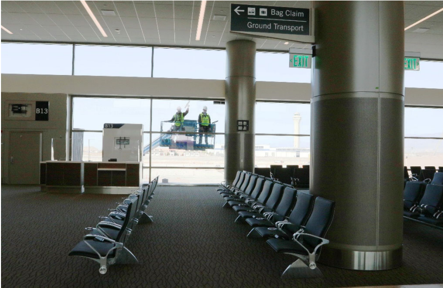
Exterior Window Cleaning
