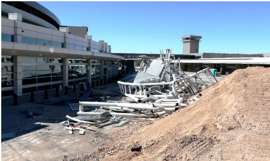
T1 Arrivals Island Canopy Demolition
