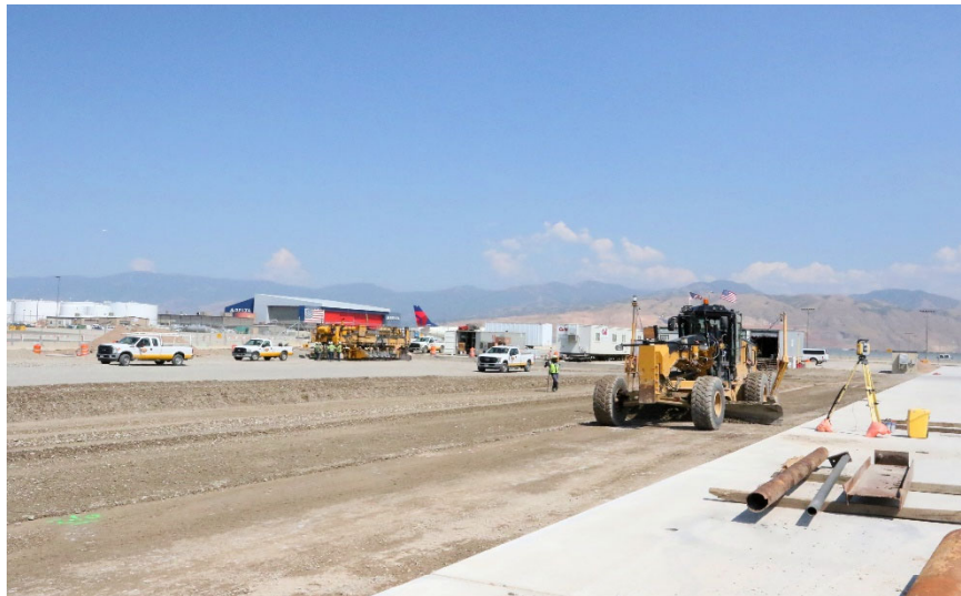
P3 Hardstand Sitework
