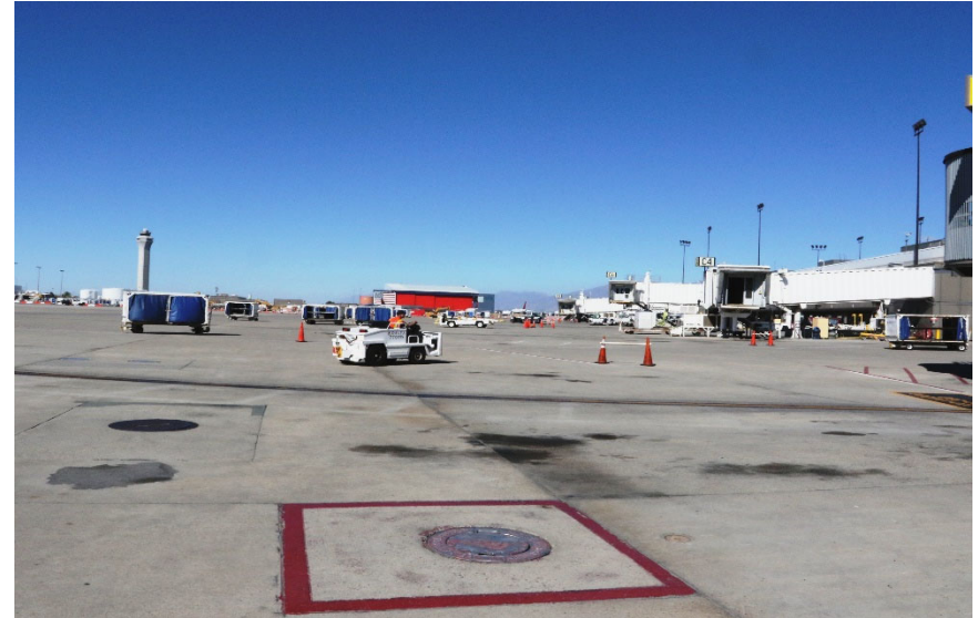
Concourse C West Gates decommissioned
