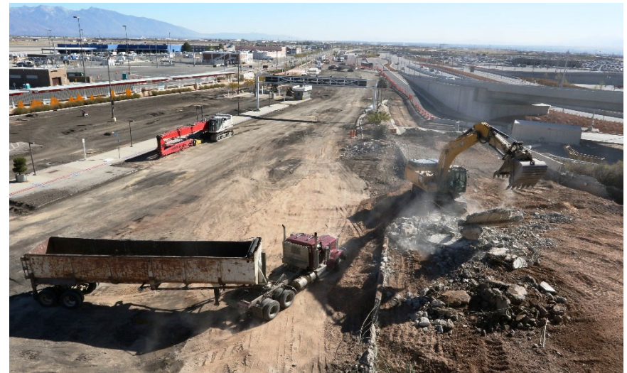
Terminal Roadways & Garage Inbound Ramp Demolition
