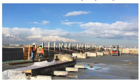
Barrier Wall formed on Parking Garage L5
