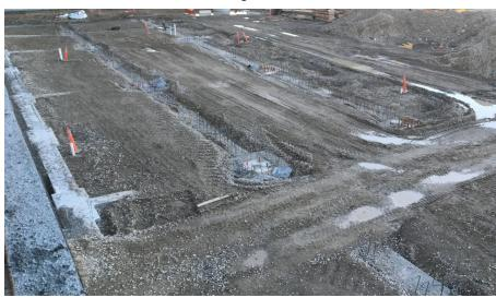
Terminal Expansion backfilled for Shallow Utilities
