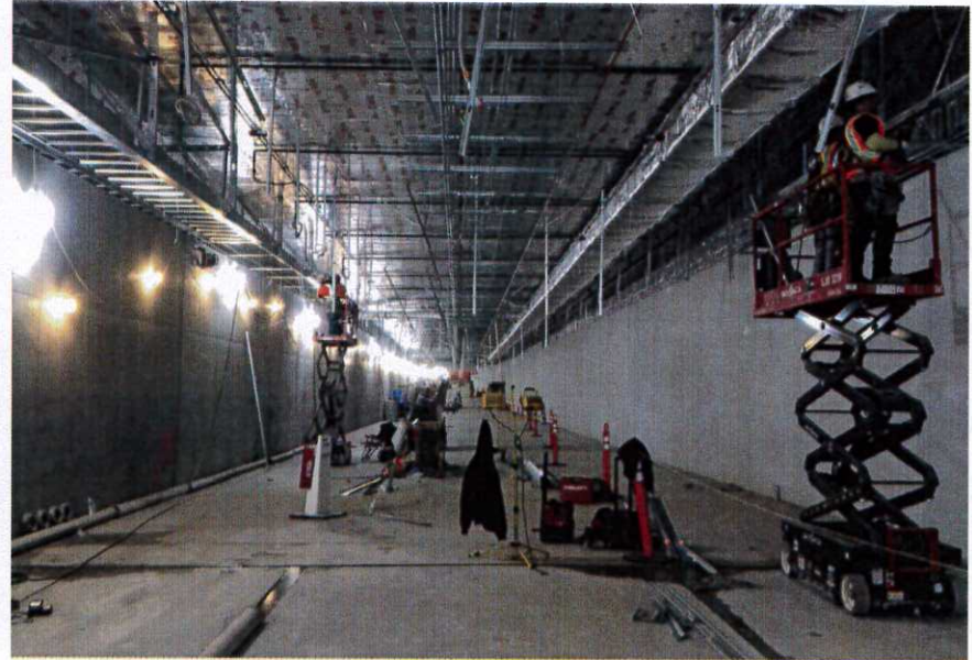
NCP Mid-Concourse Tunnel progress
