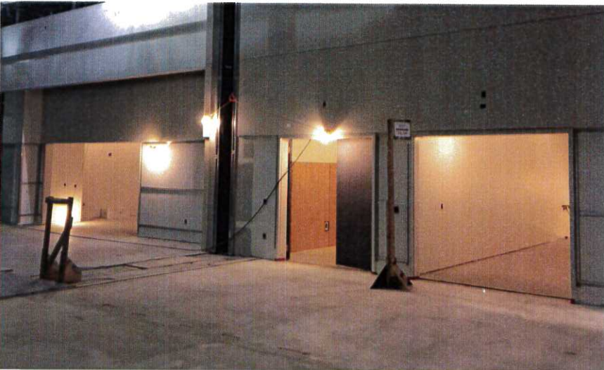
SCW Area 'F' Delta Sky Zone, Elevator and Stair Access
