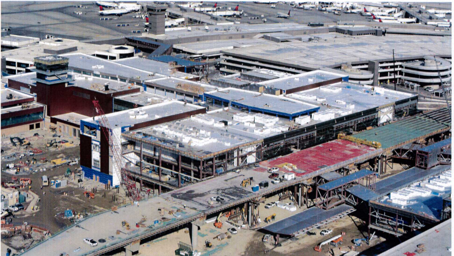
Terminal and Elevated Road looking Northeast
