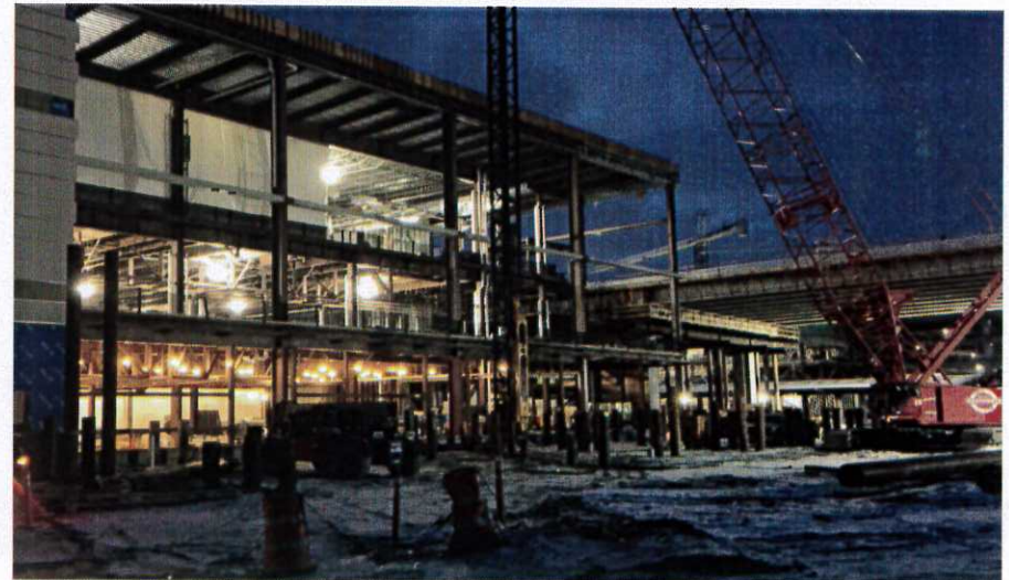
Terminal Expansion – Pile Installation
