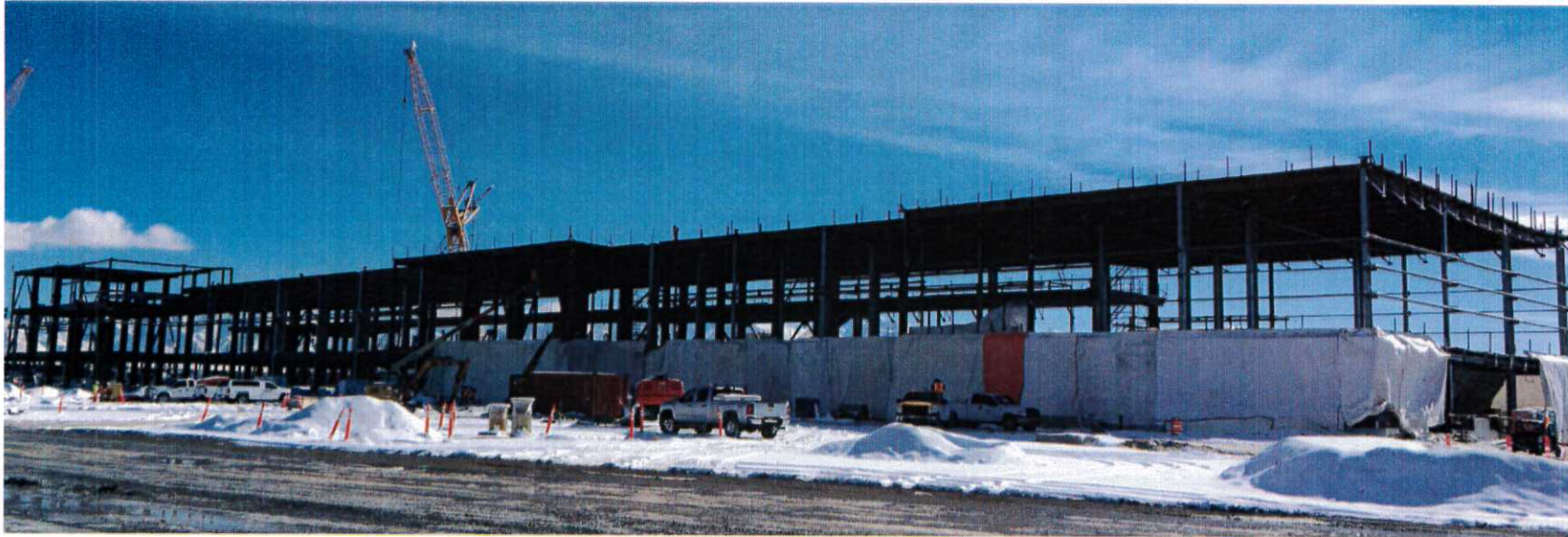
North Concourse Steel Erection looking Southeast
