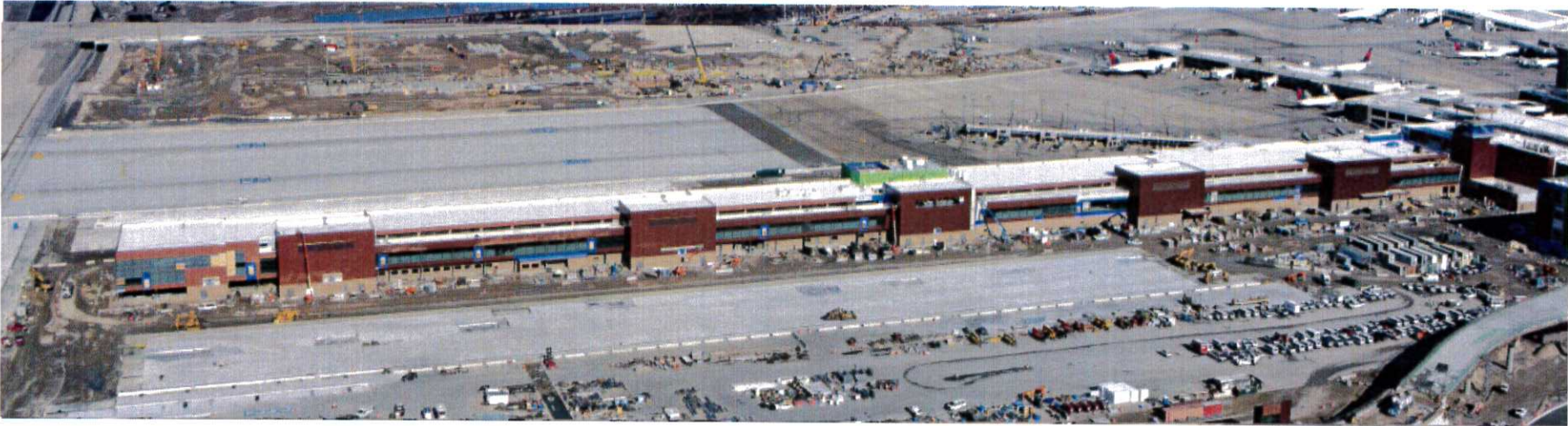
SCW Building Exterior – Areas 'A' through 'H', looking north
