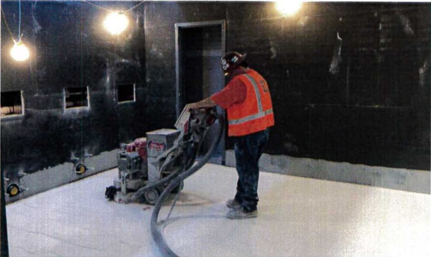
Finish grinding Terrazzo in SCW Area 'C' Rest Room
