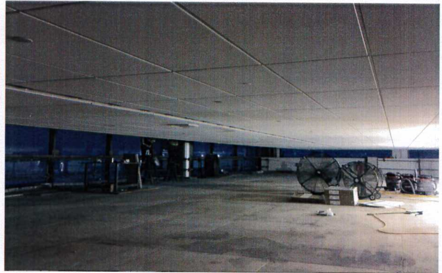
Ceiling Tile installed at Terminal Plaza High Ceiling
