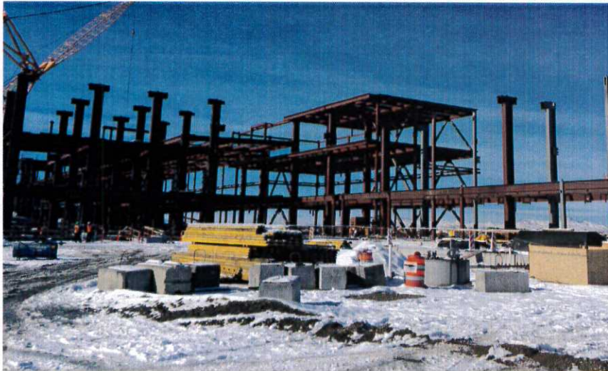
North Concourse Steel Erection Sector 'CN' and 'D'
