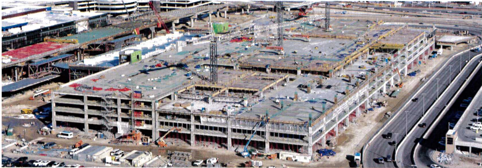
Parking Garage looking northeast
