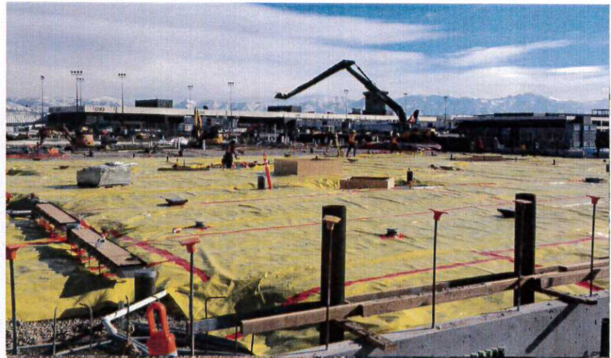
Setting up for Slab-on-Grade in NCP Sector 'E'
