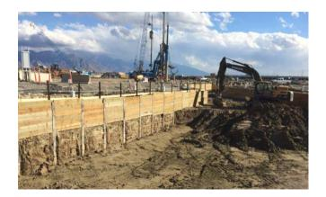
**Tunnel Excavation and Lagging Wall**
