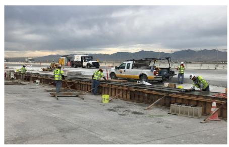
Finishing Trench Drain Pour on SCW West Apron
