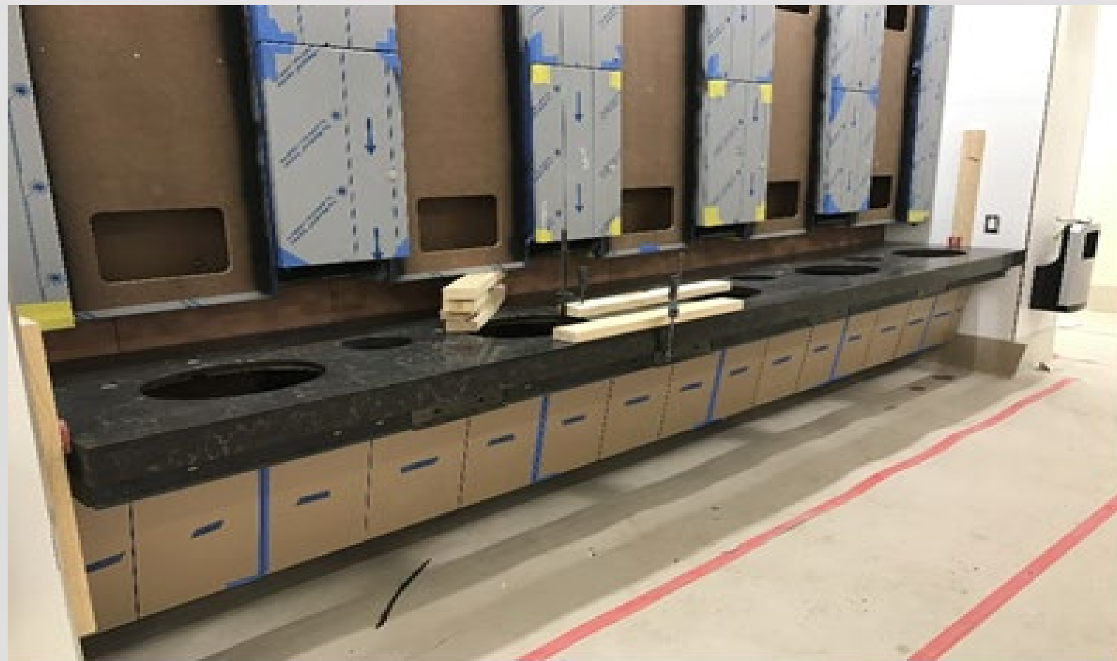
Concourse 'A' Level 2 Restroom Finishes
