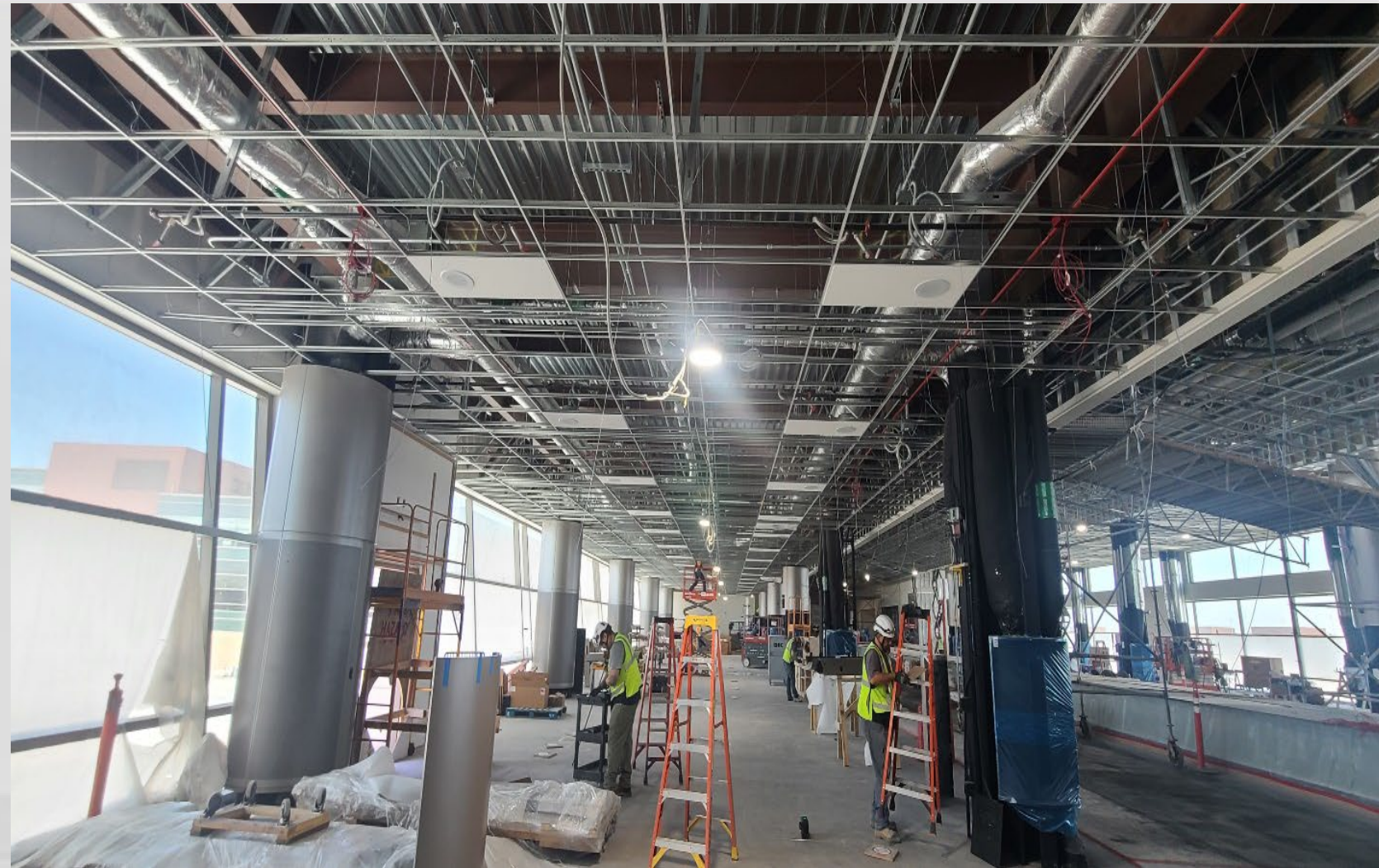
Level 2 Ceiling Grid and Column Covers
