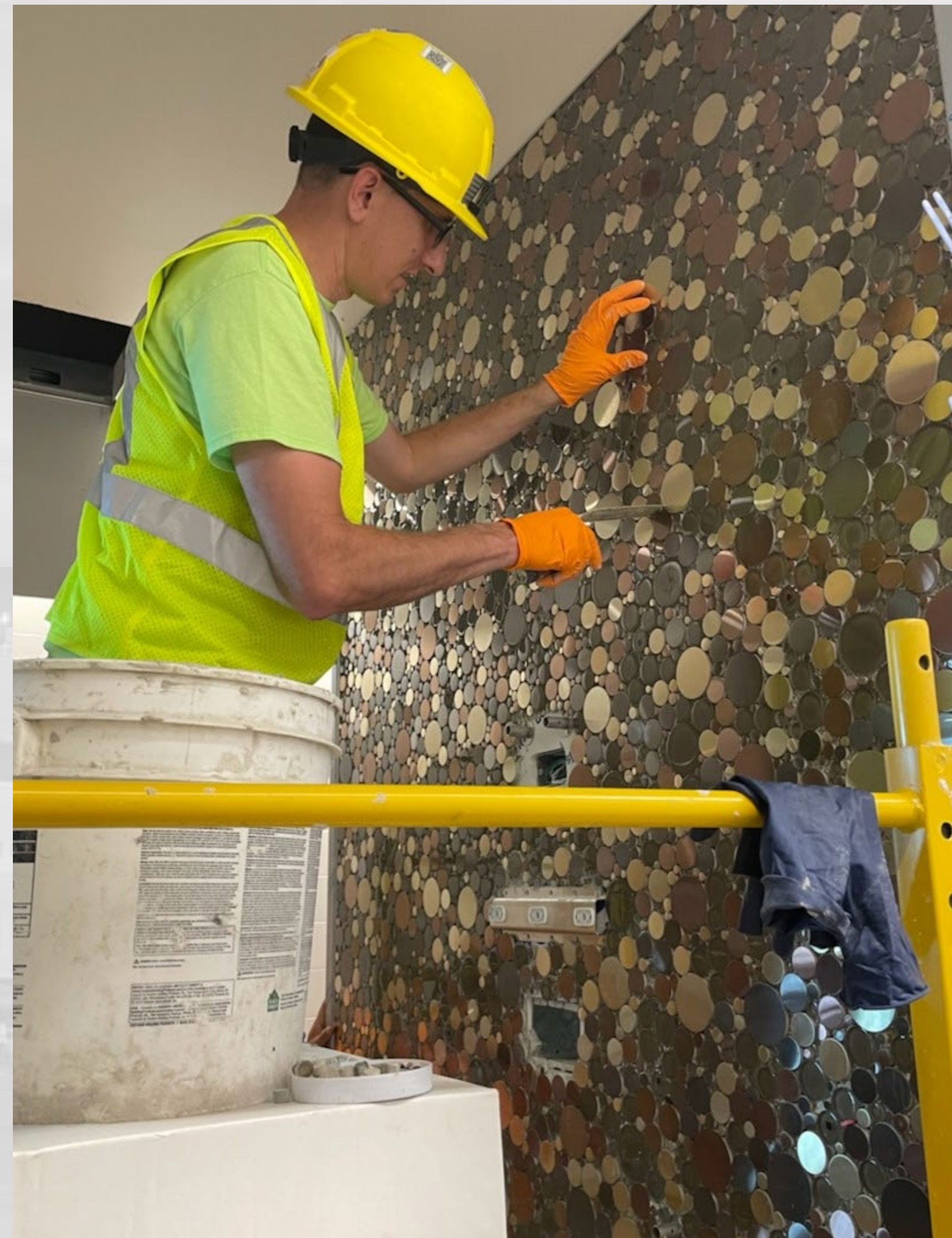
Restroom Entry Bubble Tile Installation
