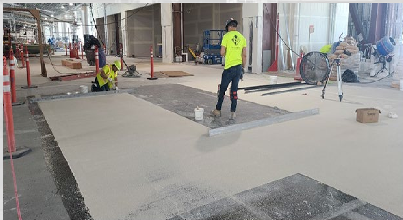
Level 2 Terrazzo Installation
