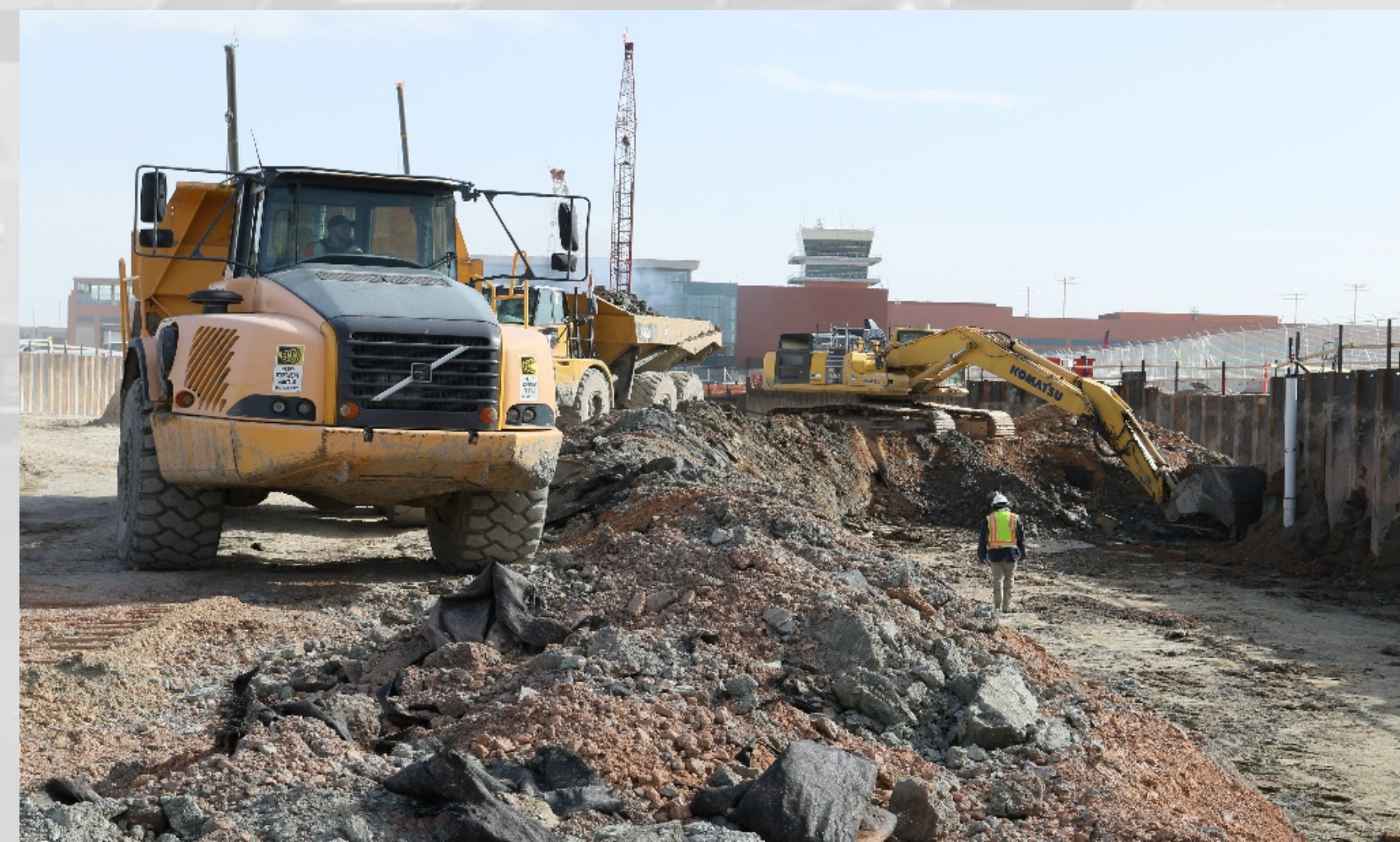
Excavation at North
