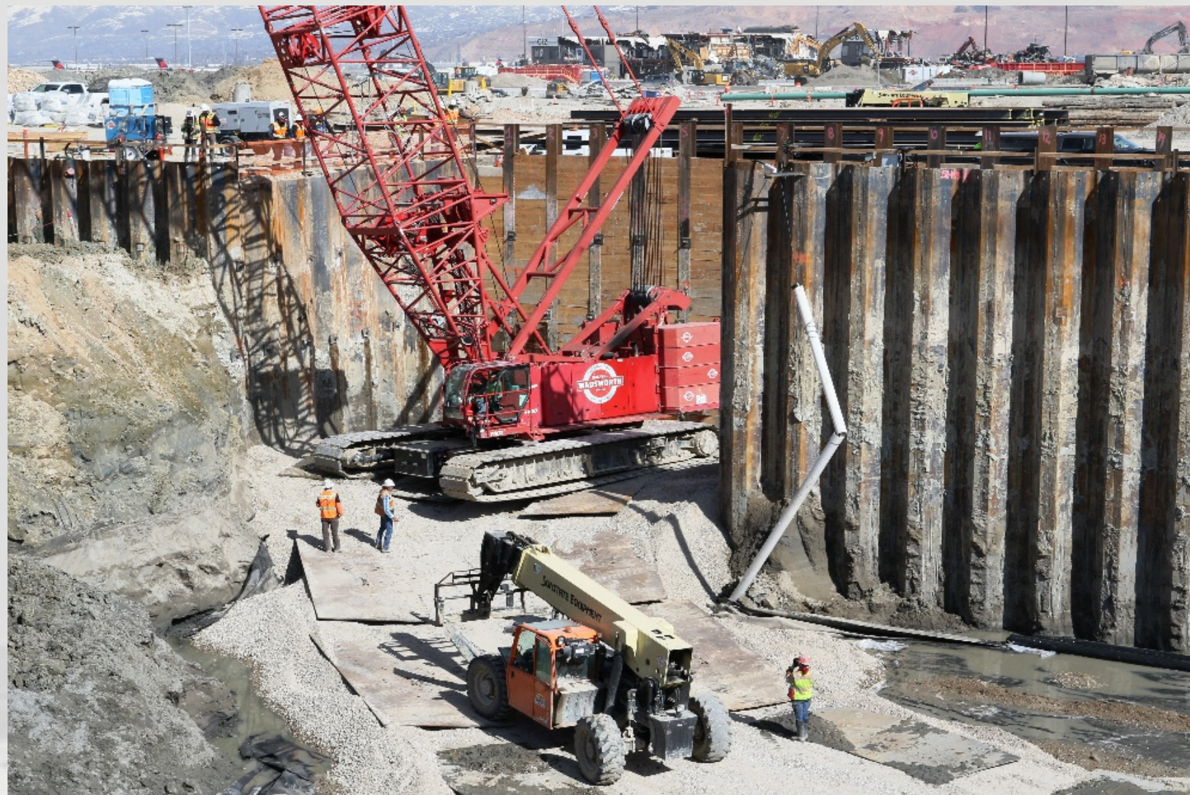
Walking Crane into Excavation
