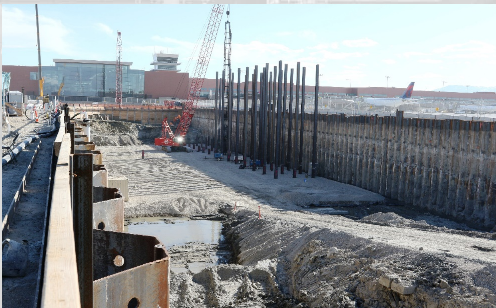
Pile Driving North End
