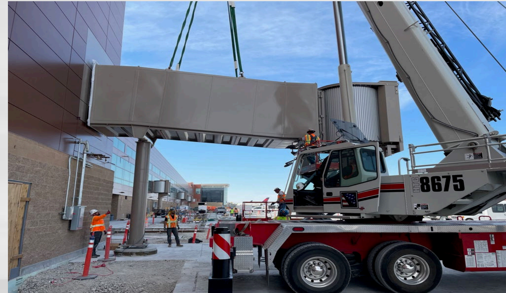
Passenger Boarding Bridge Installation
