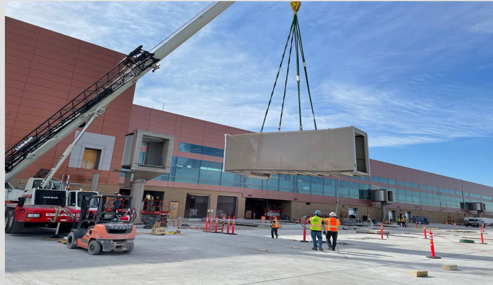
Passenger Boarding Bridge Installation
