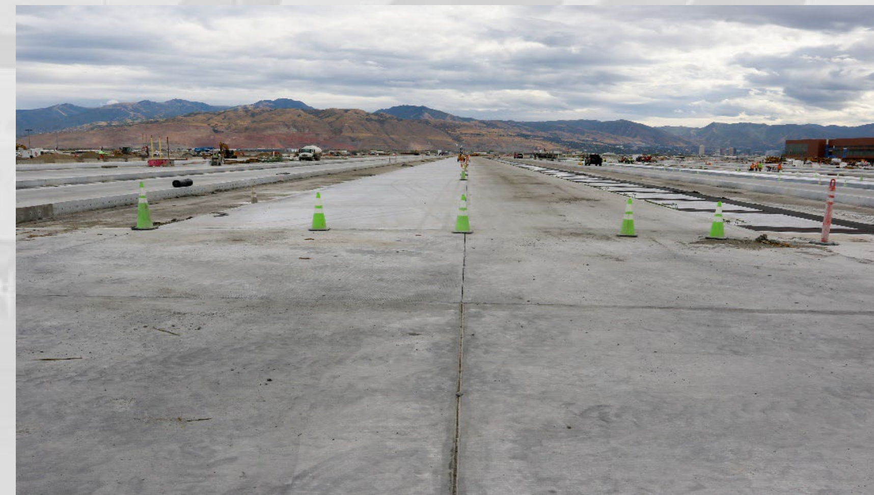
Paving Taxilane 2E Looking East
