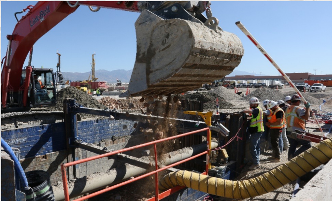
Hydrant Fuel Vault Excavation
