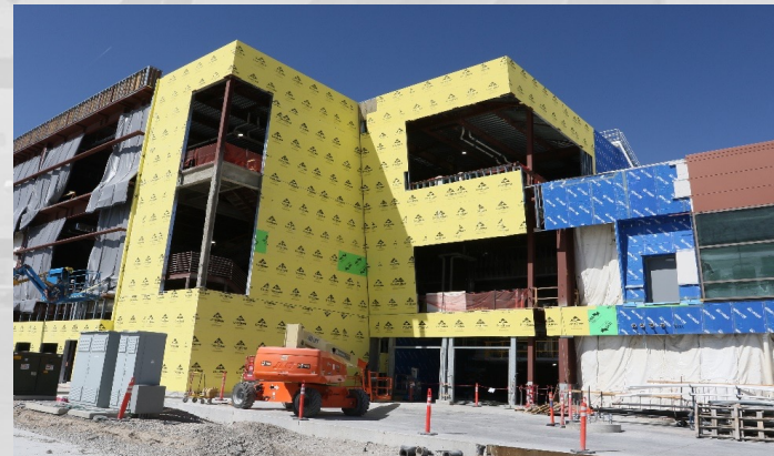
South Elevation Sheathing
