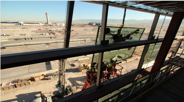
North Elevation Glass Installation
