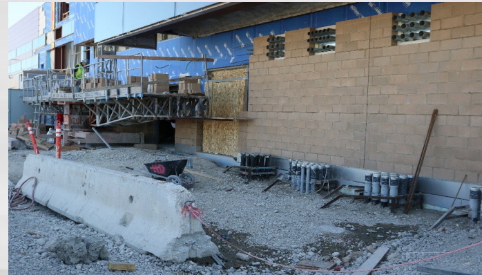
North Elevation Masonry Installation
