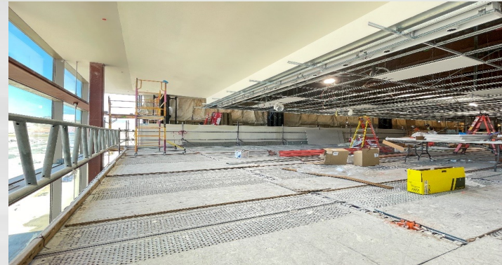
Canyon High Ceiling Finishes and Grid
