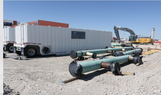
20" Fuel Line Relocation Flushing Prep
