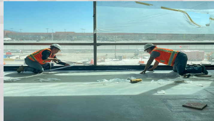
Level 2 Interior Glazing Trim
