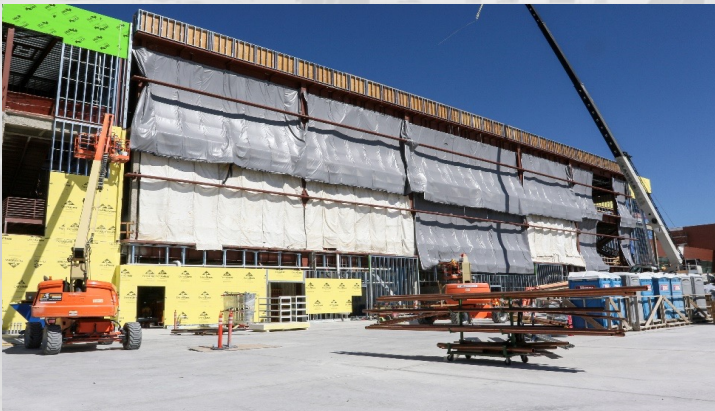
South Elevation Temporary Dry-in
