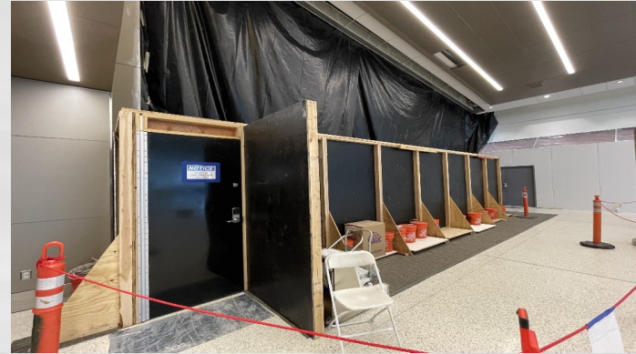
Level 2 Temporary Barricade
