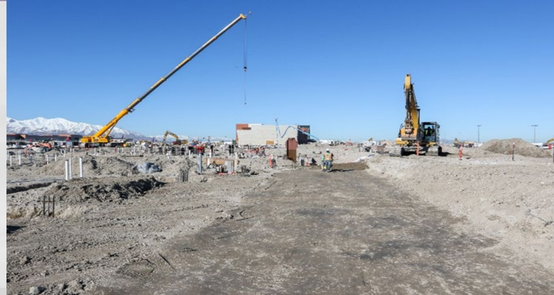
North Ductbank and Backfill
