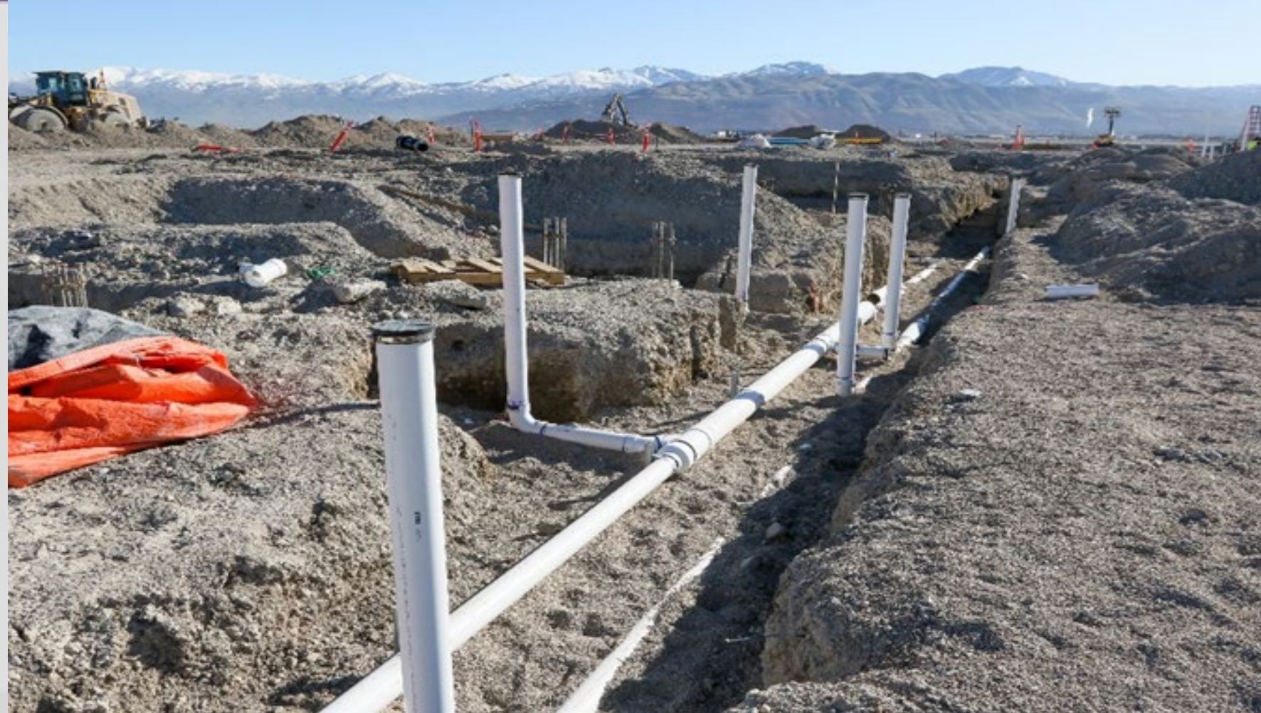
Underground Plumbing Installation
