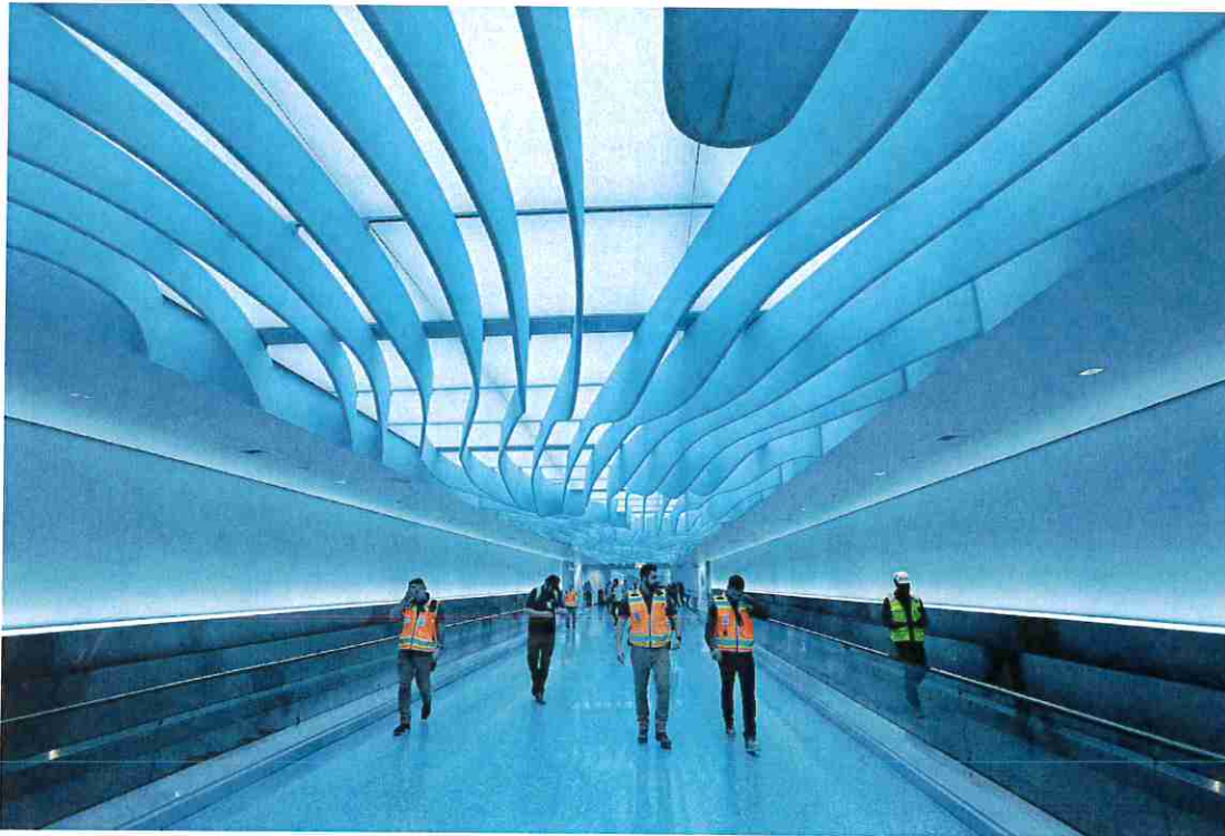
Construction workers walk through the completed Salt Lake City International Airport's River Tunnel in Salt Lake City on Wednesday, April 3, 2024. | Jeffrey D. Allred, Deseret News
