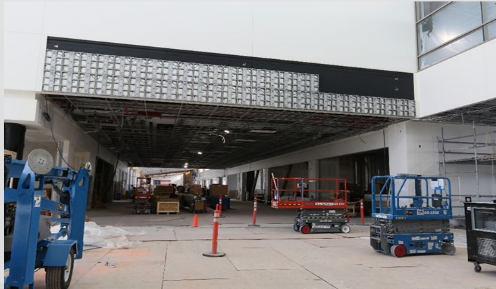
Dynamic Sign Installation
