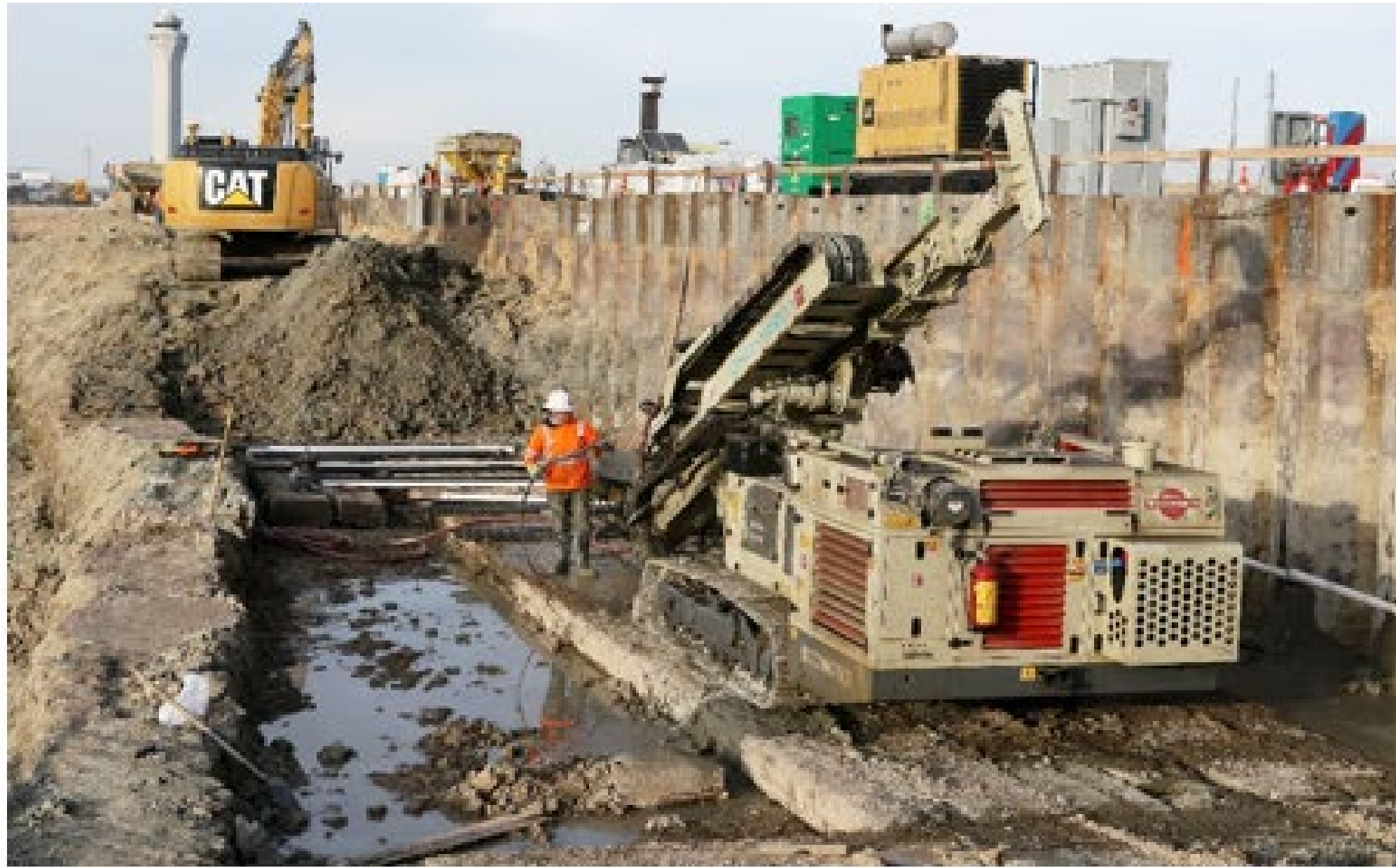
Central Tunnel Tie-Back Installation
