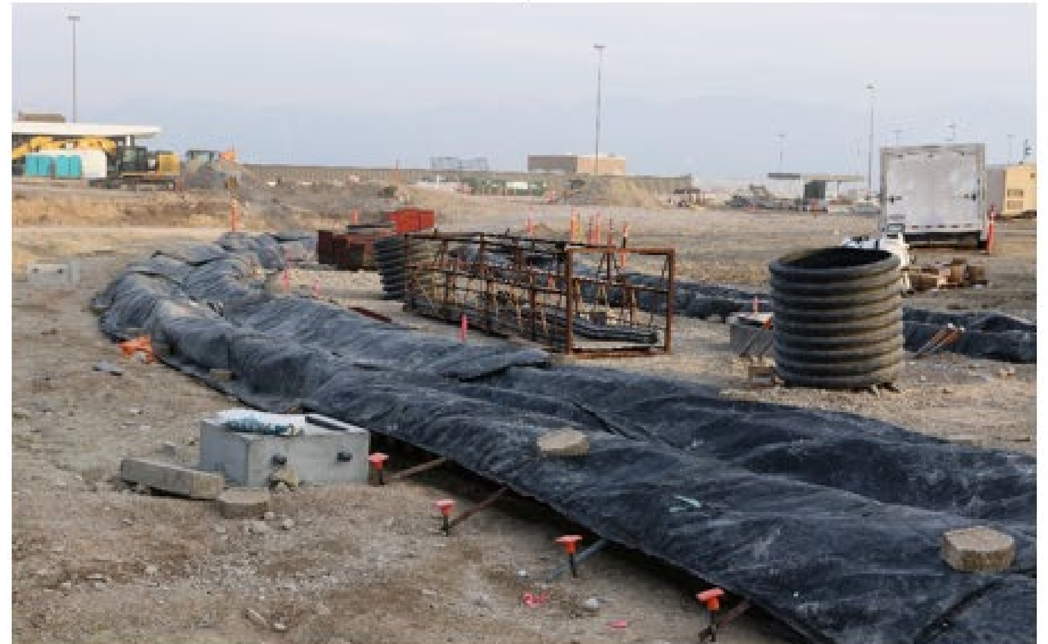
TRAX Track Installation Looking Southeast
