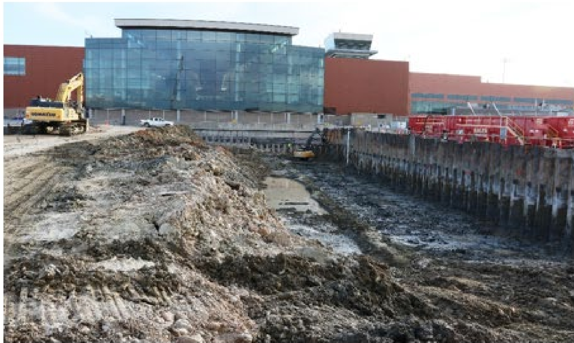
Central Tunnel Excavation Looking South - Mid-January
