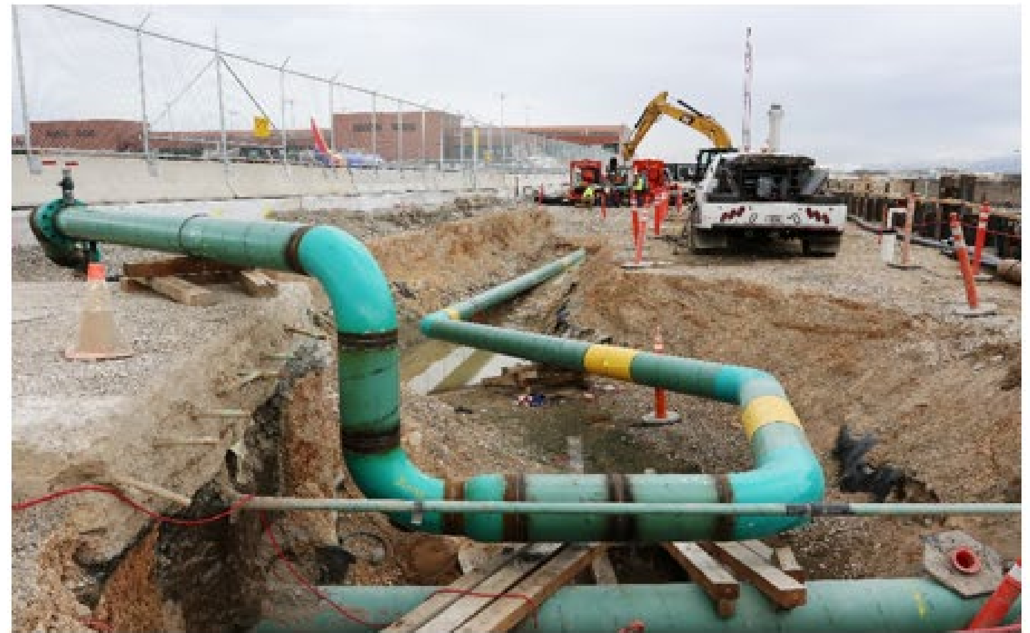
Fuel Line Installation Adjacent to Central Tunnel
