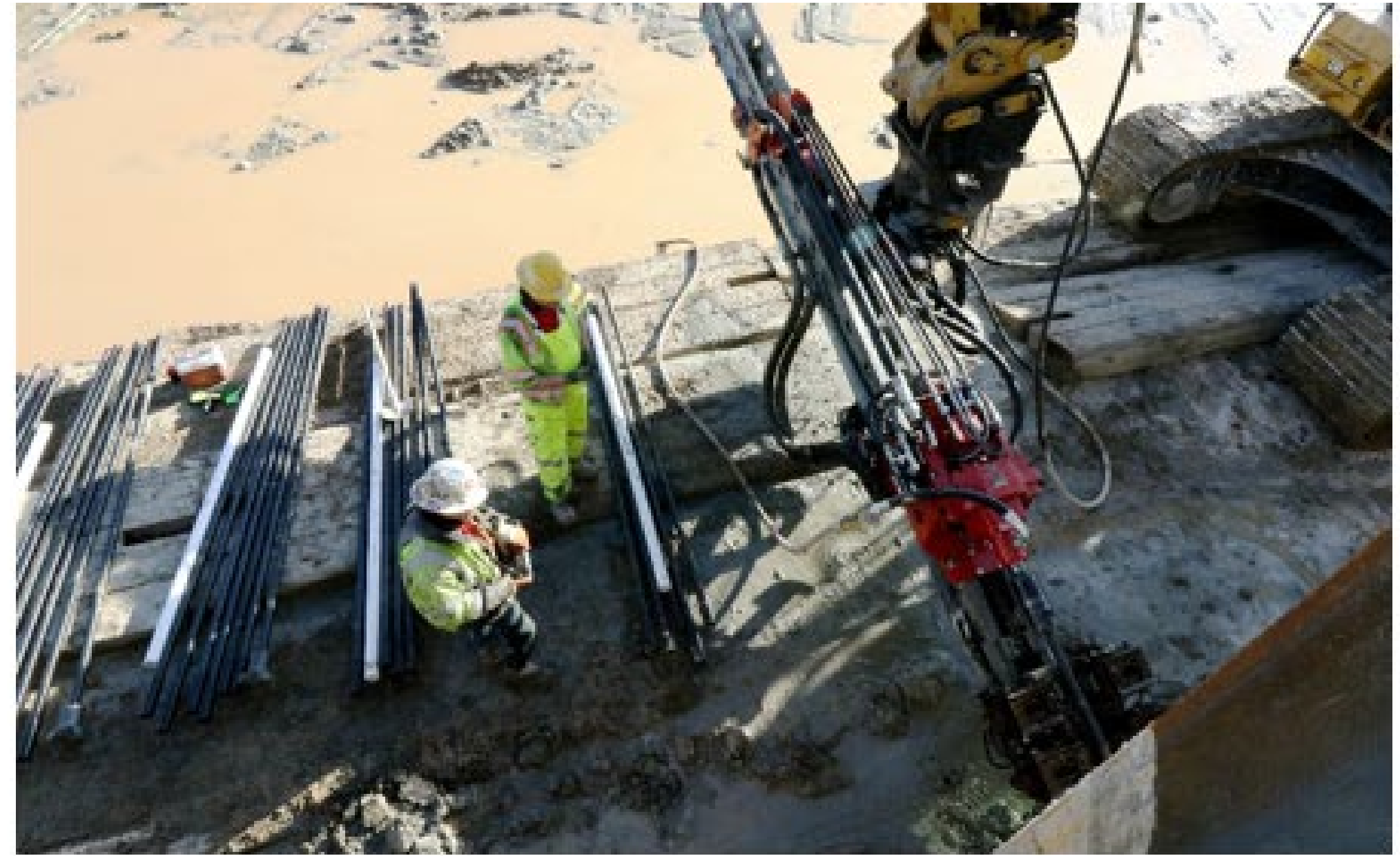
Central Tunnel Tie-back Installation
