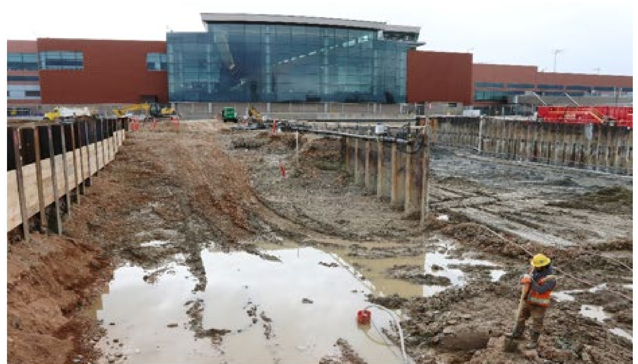
Central Tunnel Excavation Looking South - End of January
