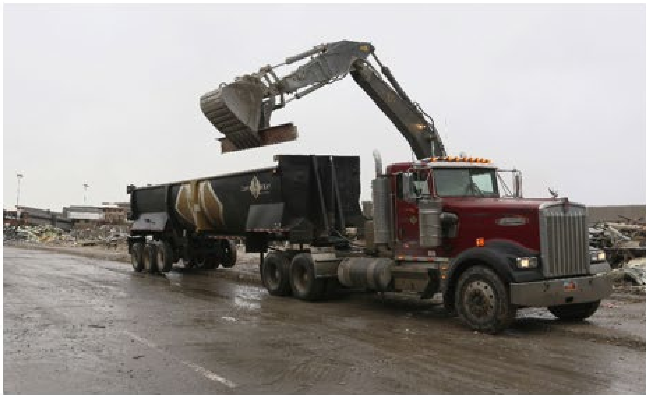
Demolition Rubble Loading at Terminal 1
