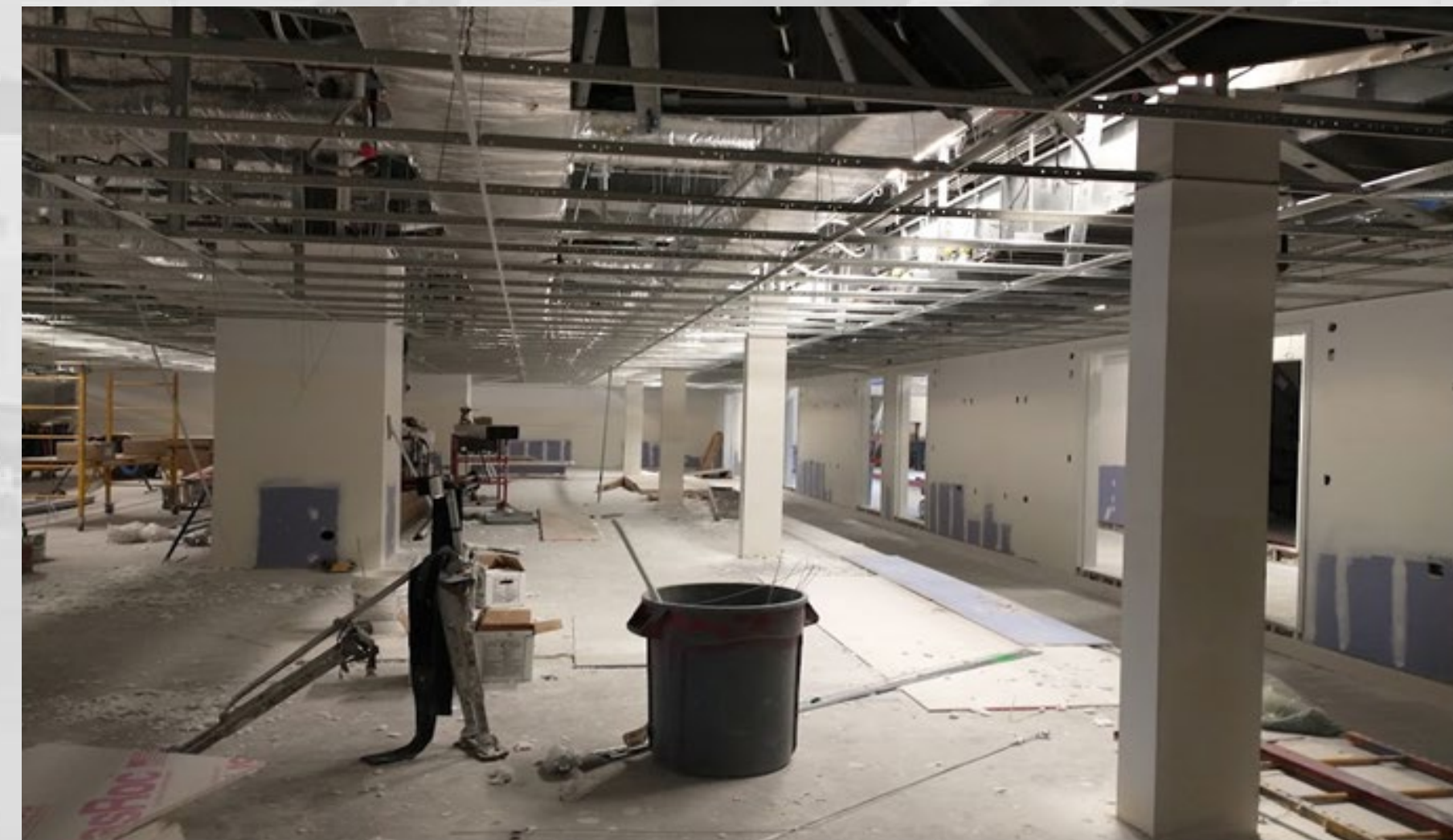
Level 1 Ceiling Grid and Wall Finishing
