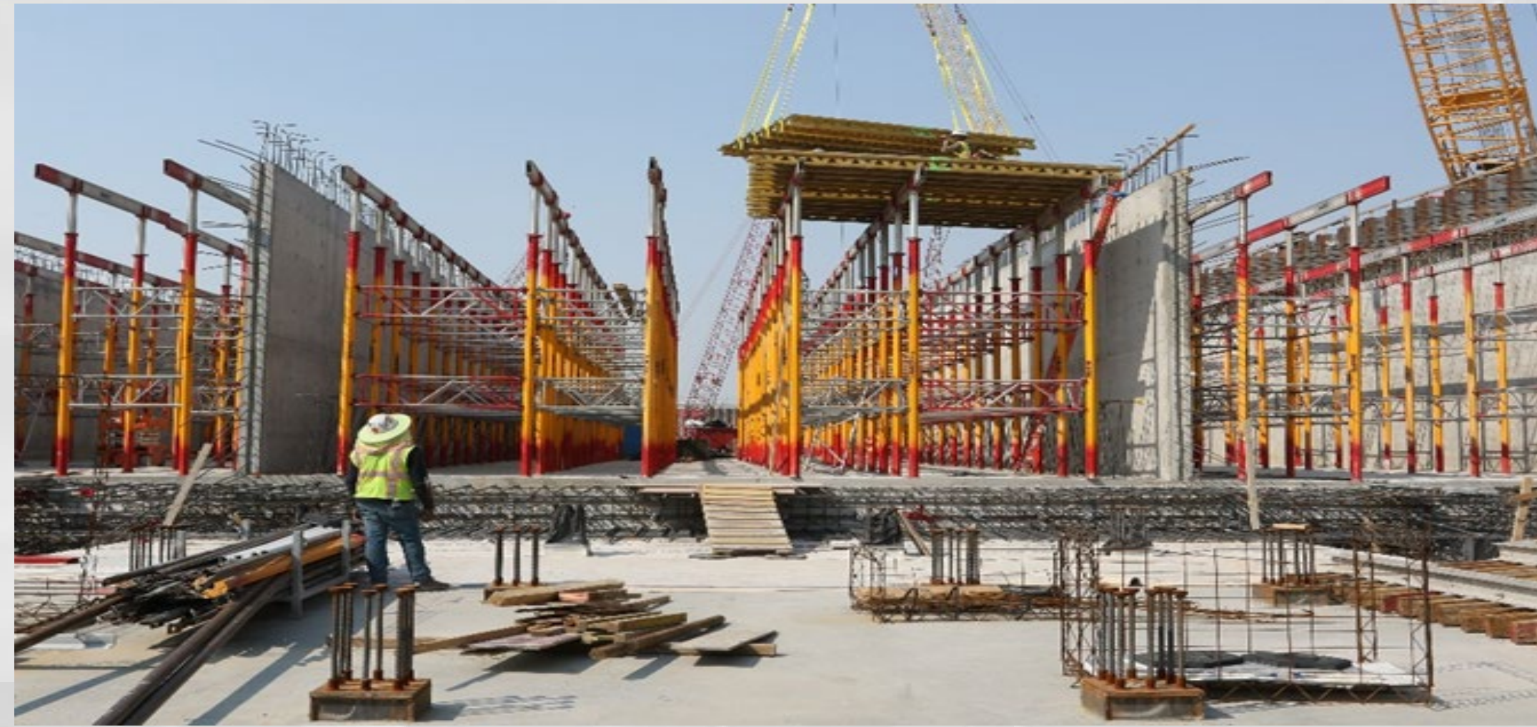
Wall and Lid Formwork
