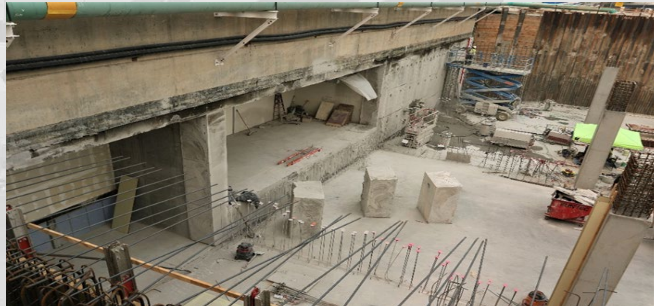
Terminal Basement Concrete Wall Removal
