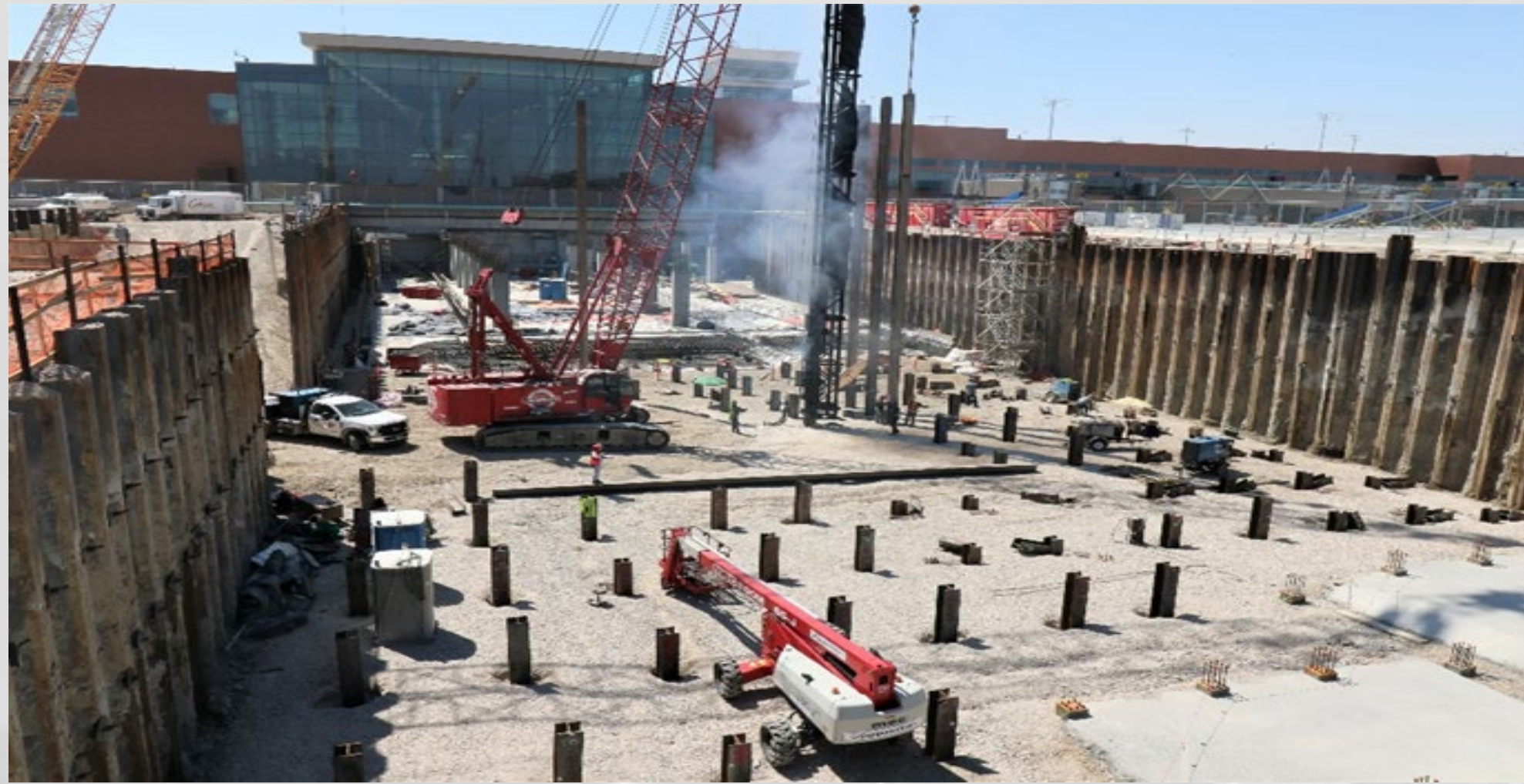
Temporary Fuel Line Area – Final Pile Driving
