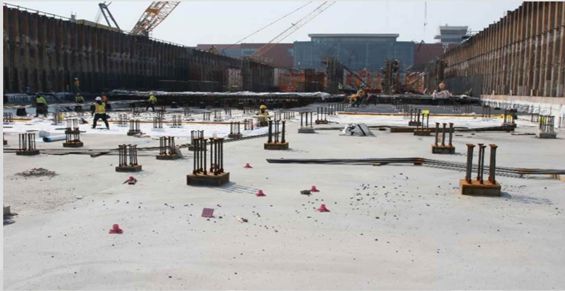
Mud Slab and Waterproofing
