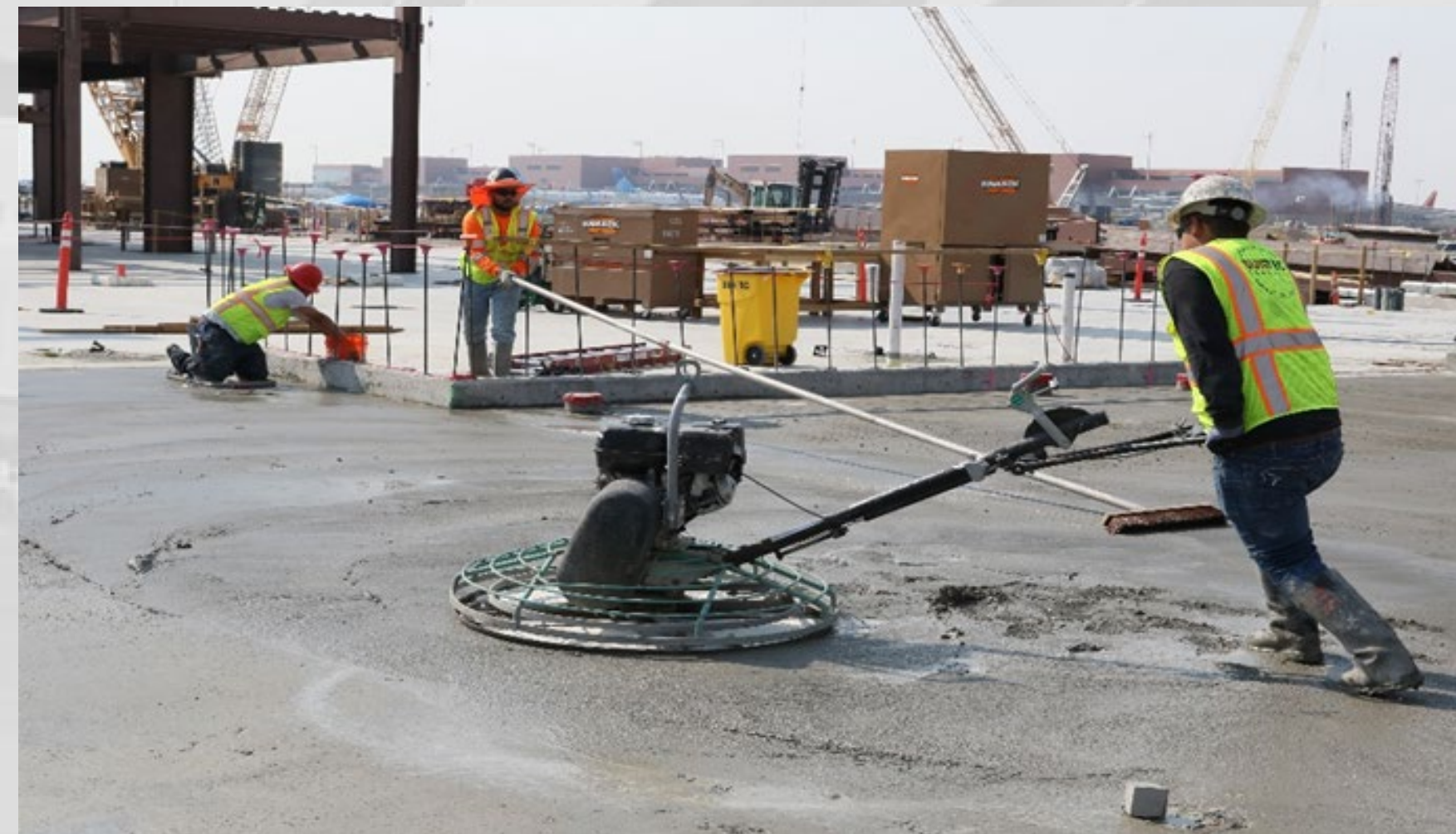
Area 'C' Drive-thru Concrete Finishing
