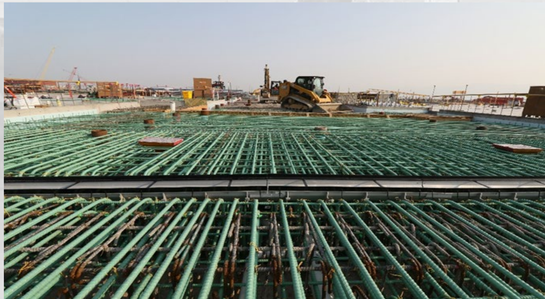
Area 'C' Drive-thru Epoxy Coated Rebar
