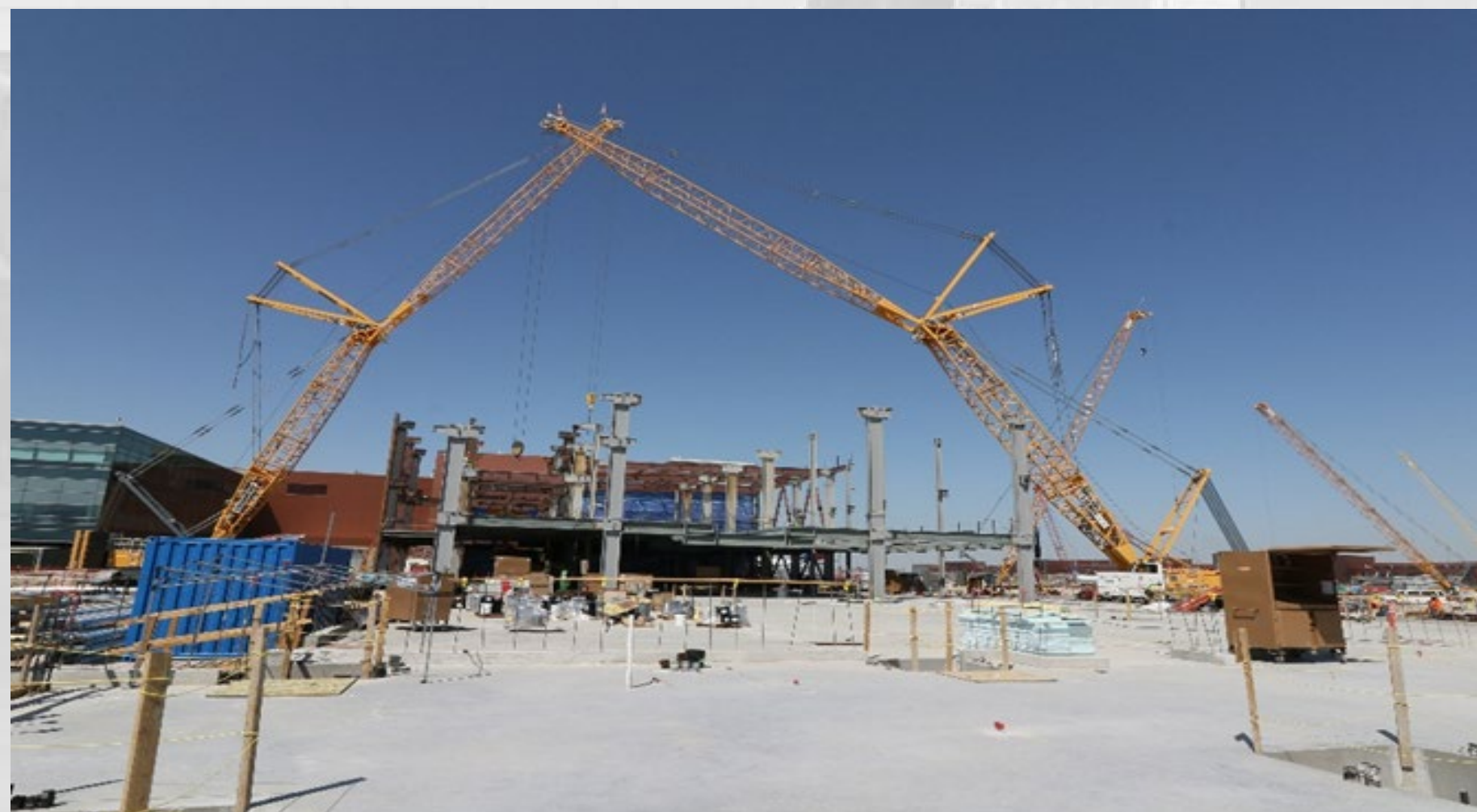
August 12 – Steel Erection Progress
