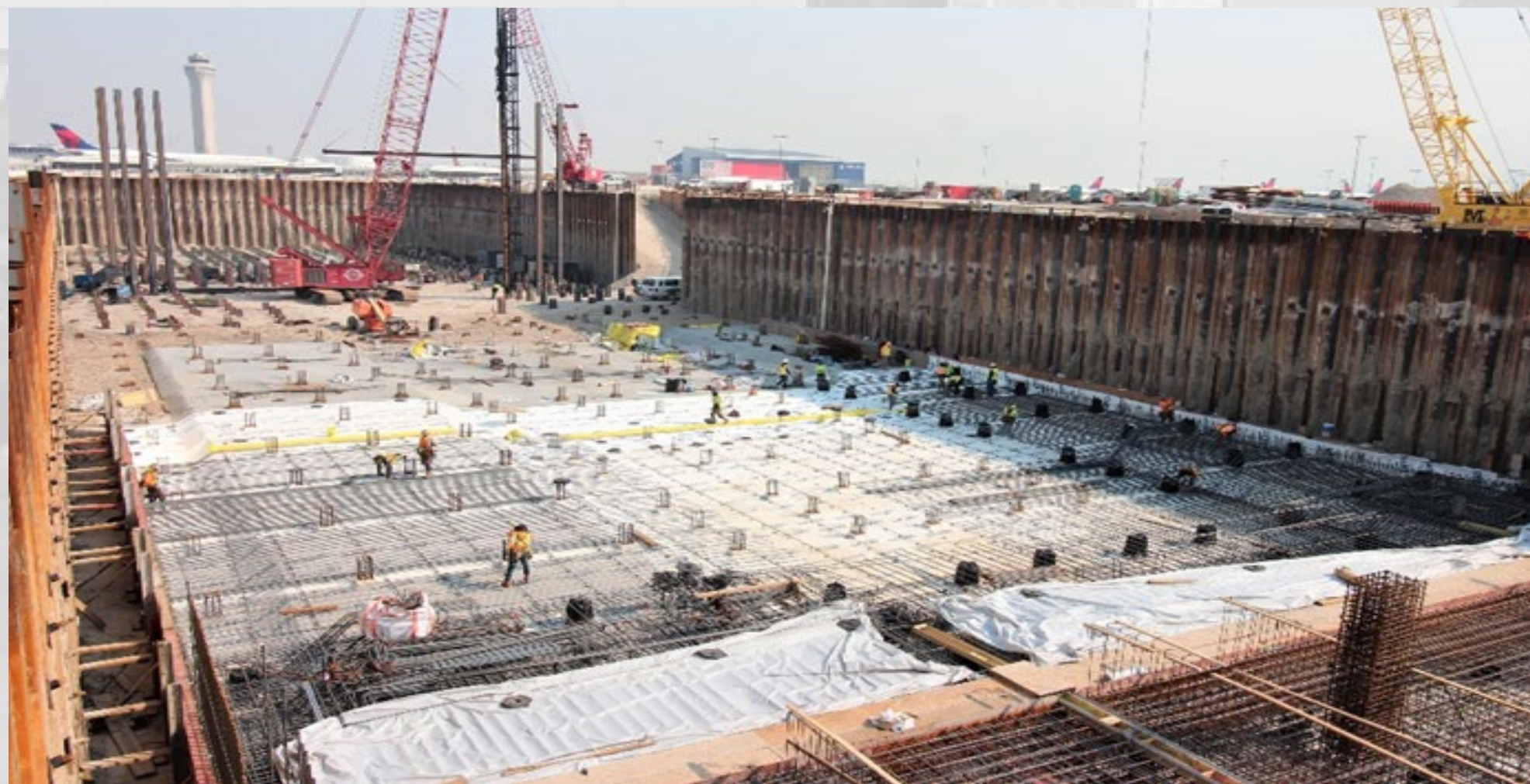
Mat Slab Formwork
