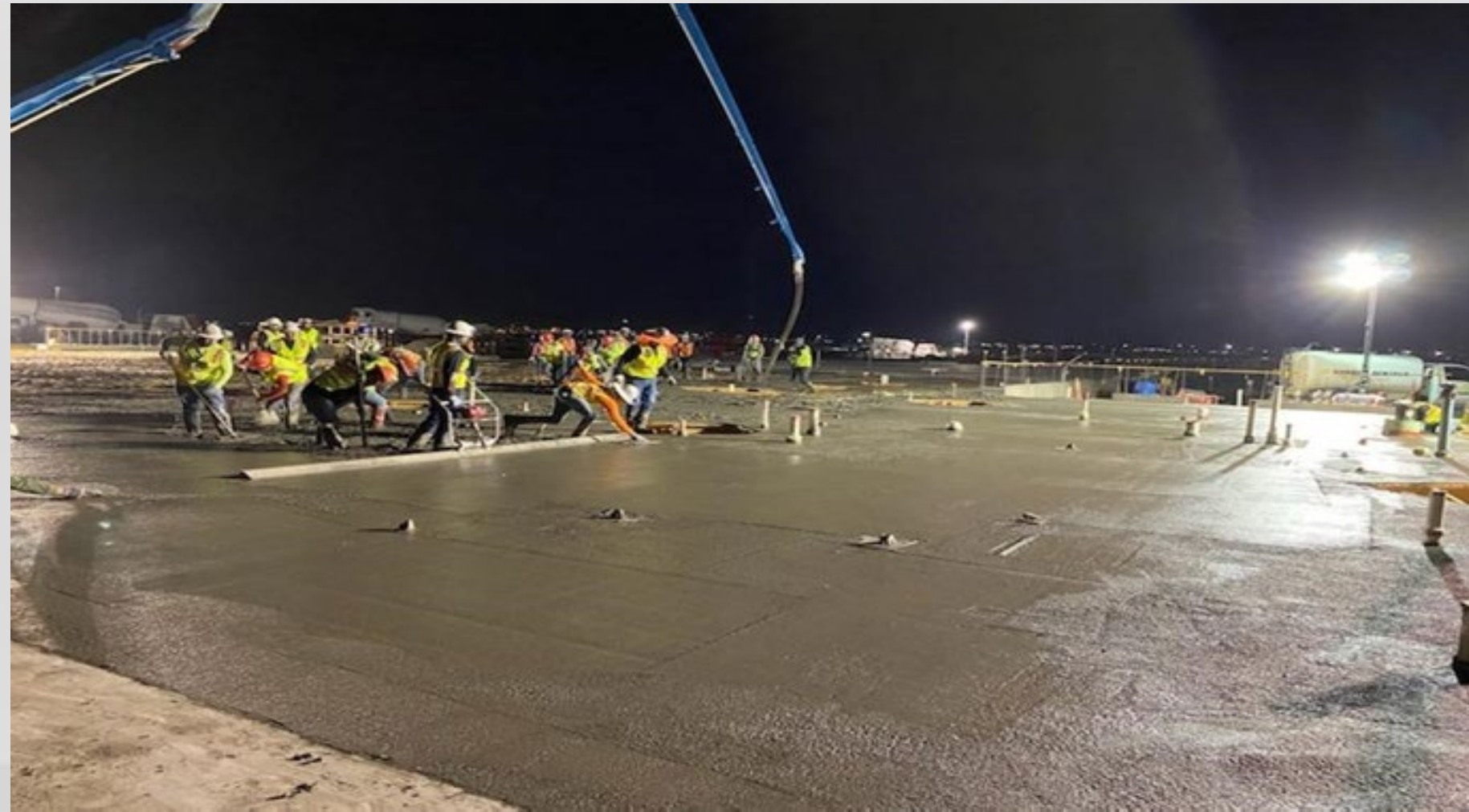
Area 'D' Slab-on-Grade Concrete Placement
