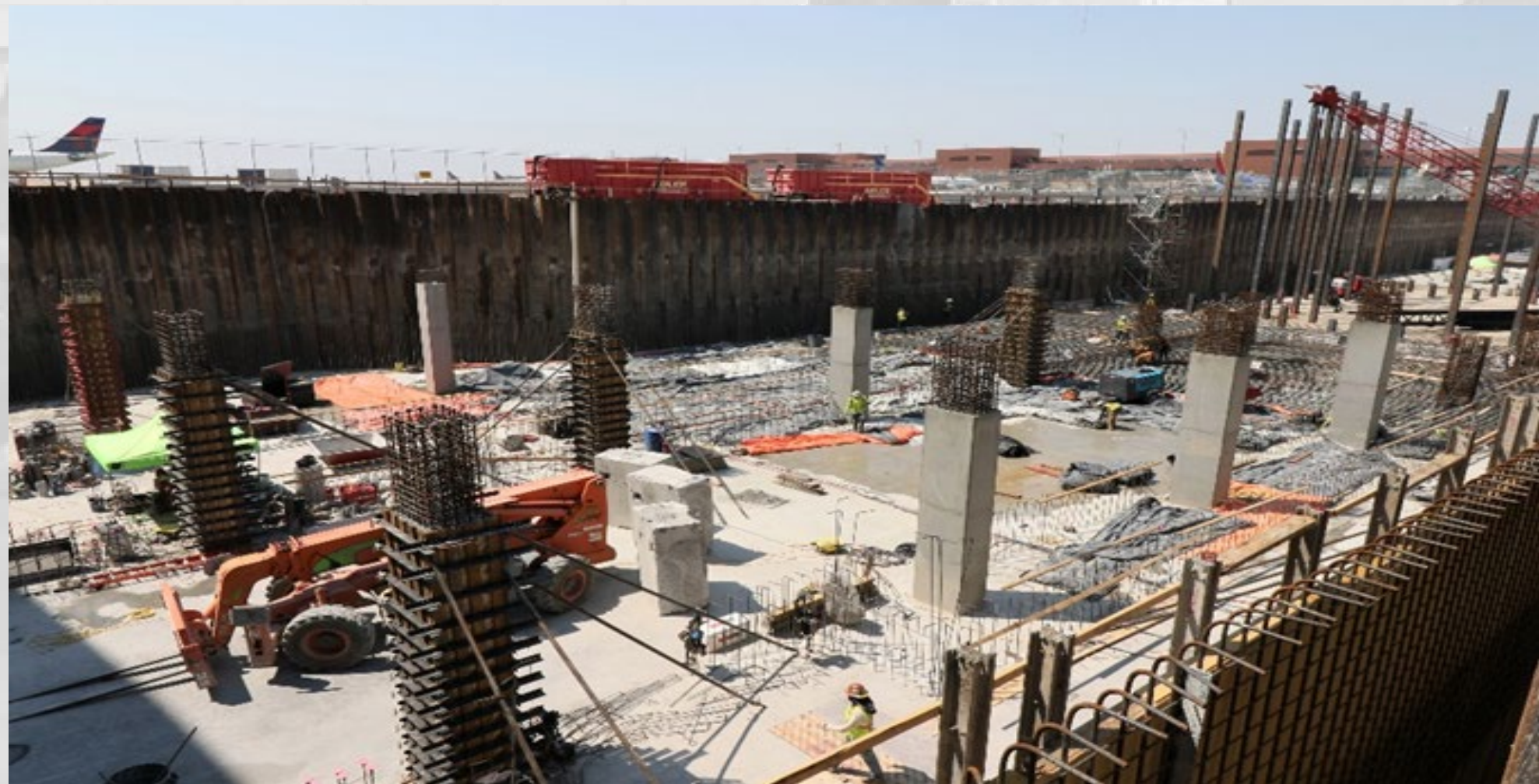
Column and Wall Formwork
