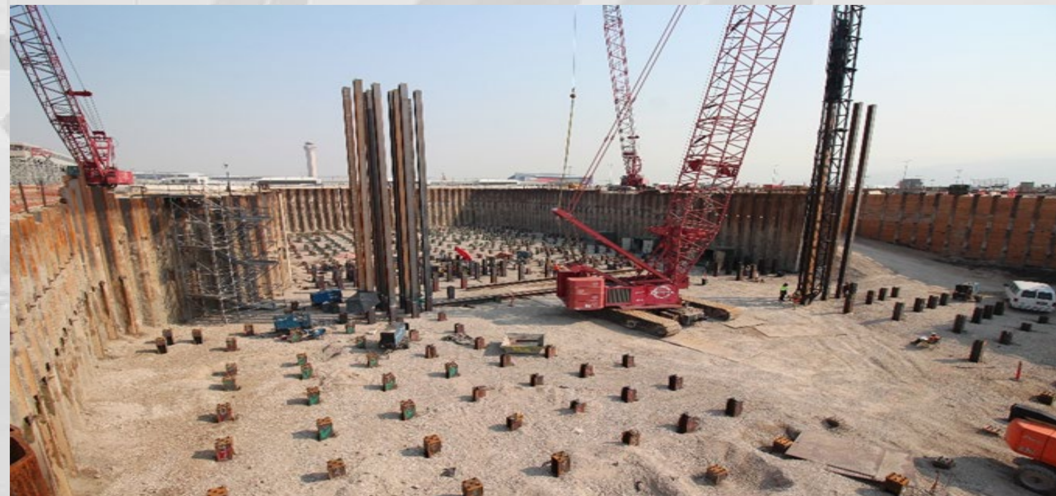
Concourse 'B' Node Basement Pile Driving
