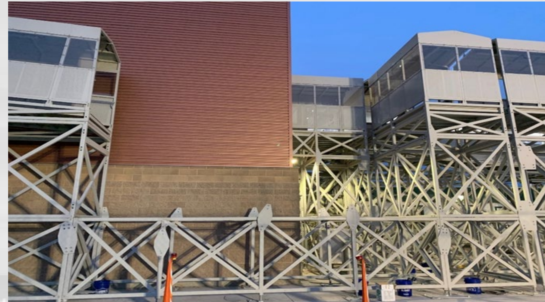
Exterior Ramp Installation
