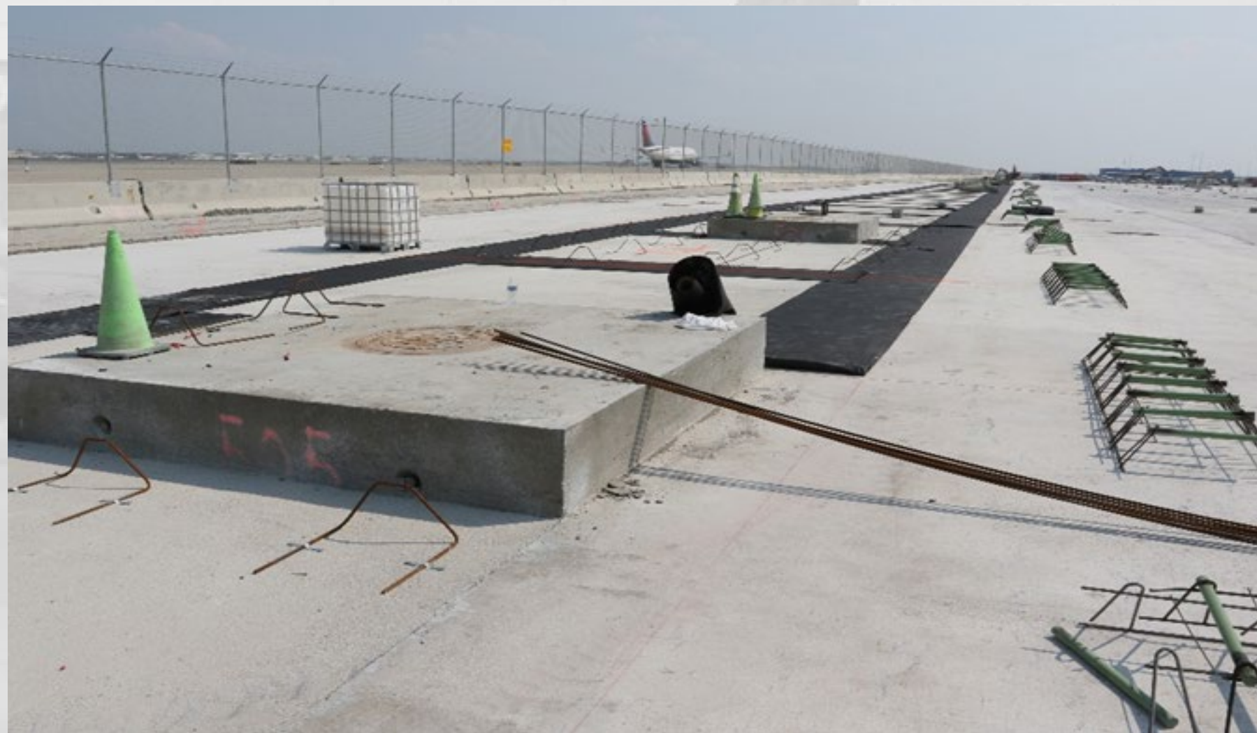
Airfield East (Near Runway) Paving Prep
