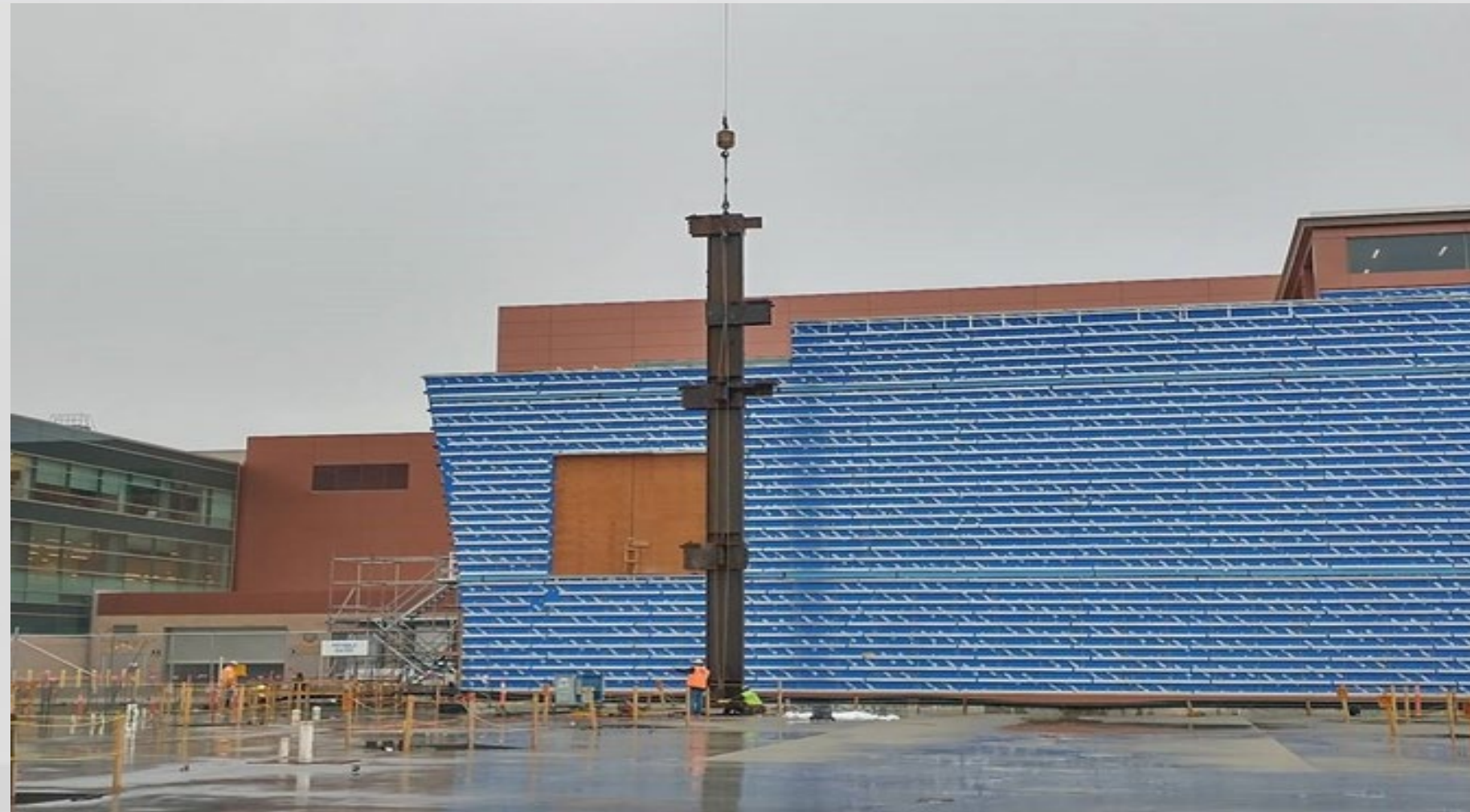
August 2 – Day One Steel Erection
