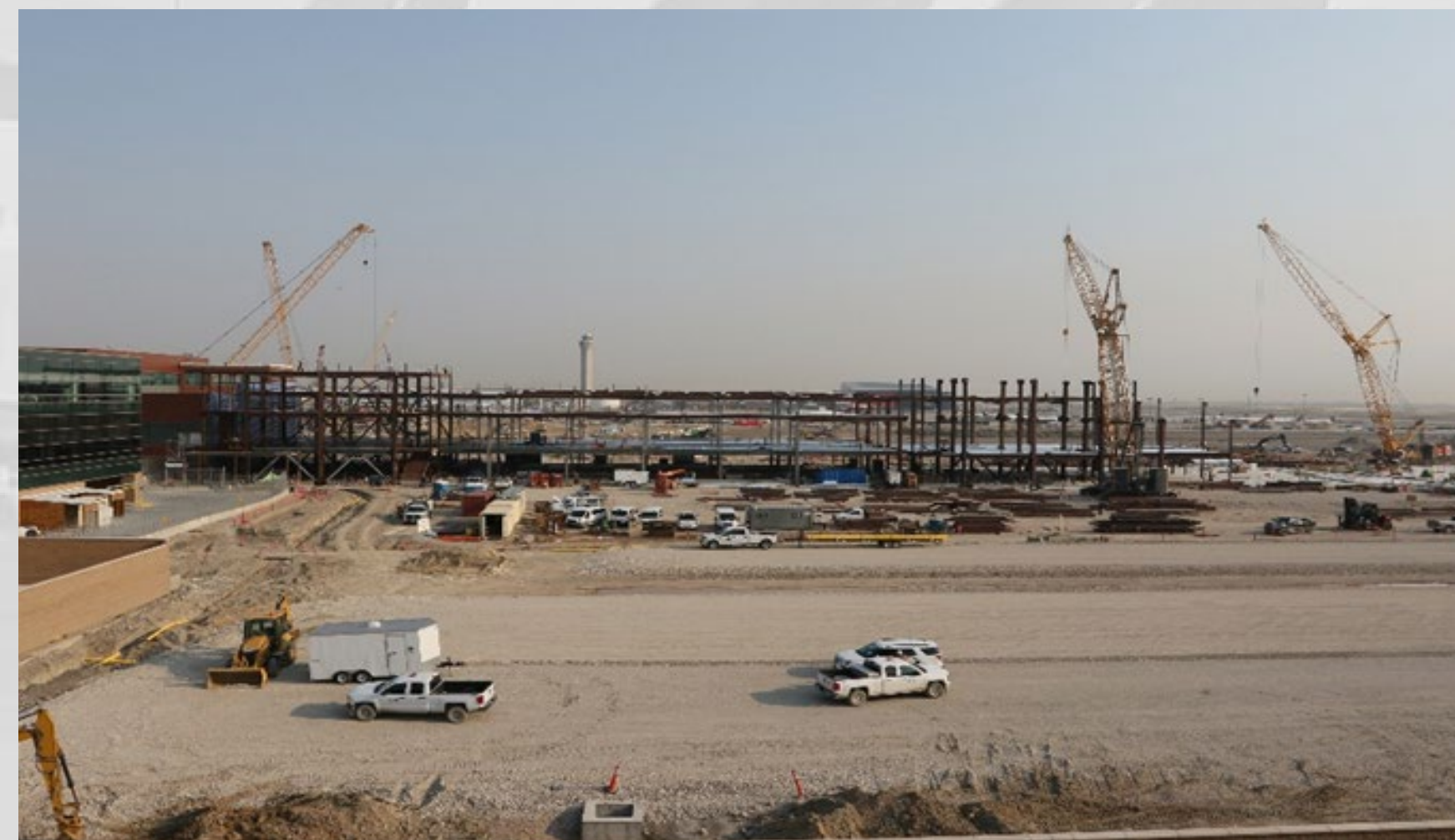
August 27 – Steel Erection Progress
