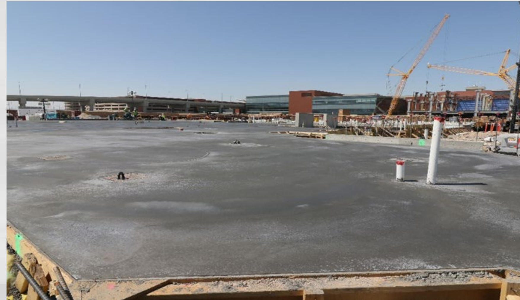
Area 'D' Slab-on-Grade Finished Concrete
