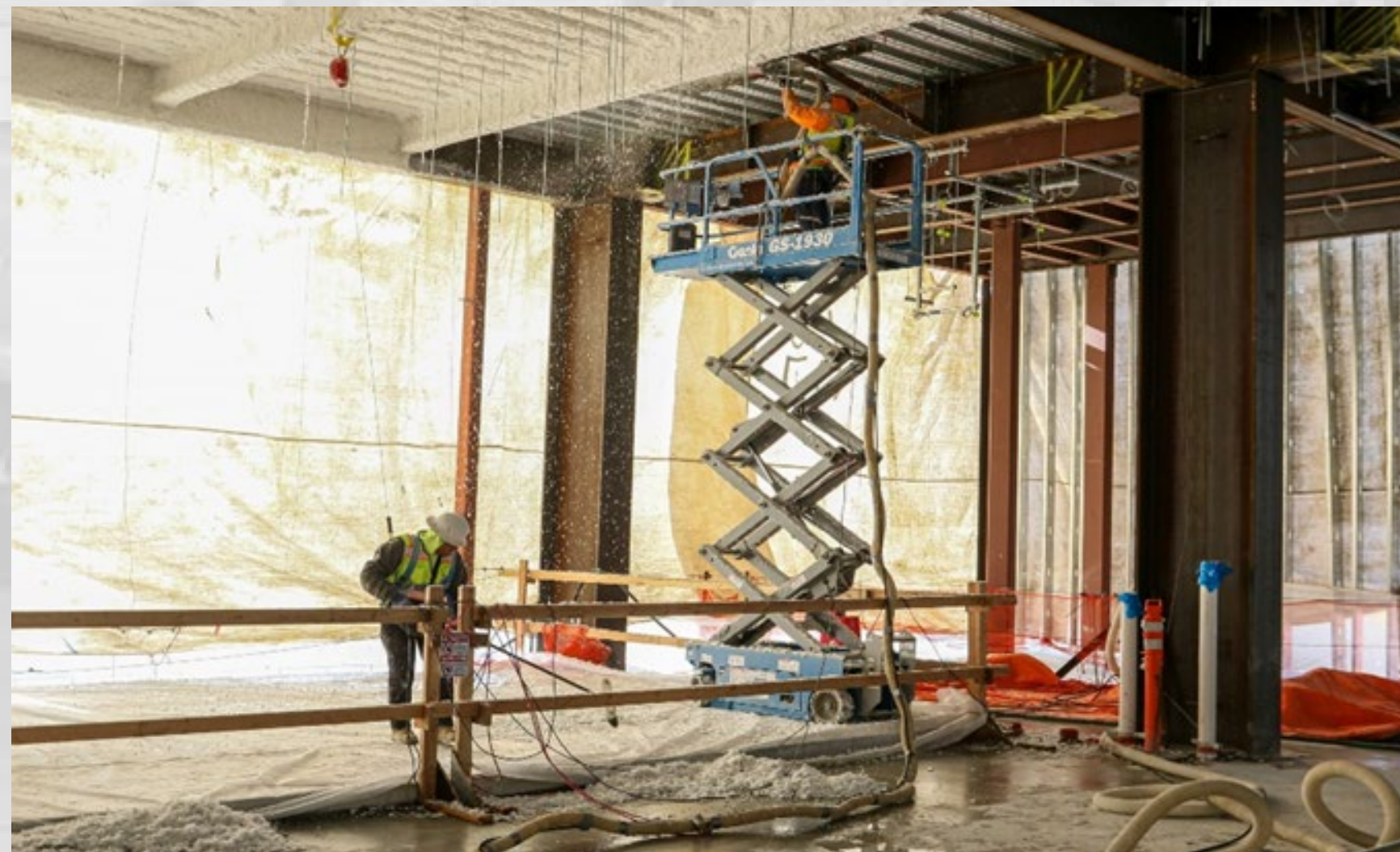
Area H Level 3 Spray Fireproofing
