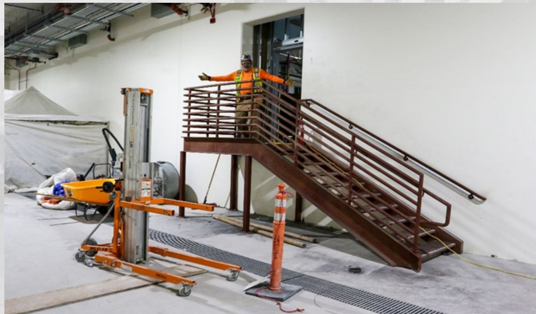
Stairs into APM Cell
