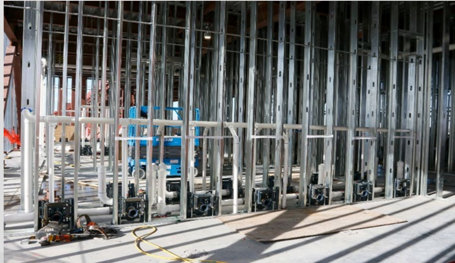
Public Restroom Studs and Carriers
