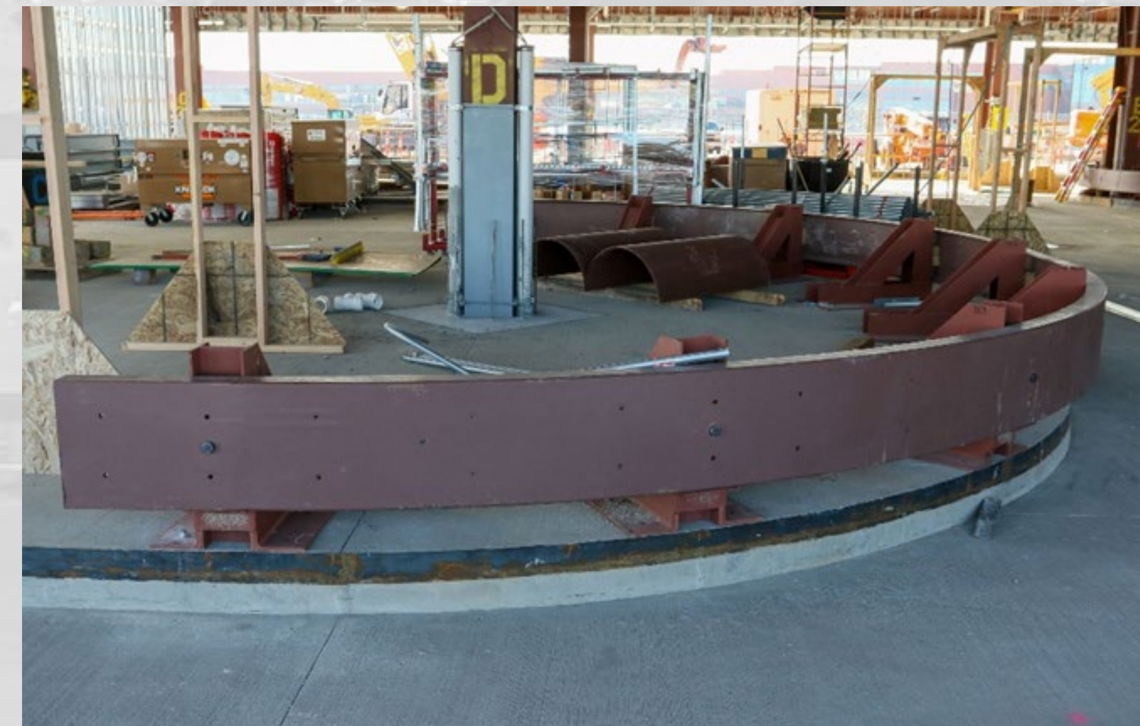
Area J Baggage Make-up Carousel Protection
