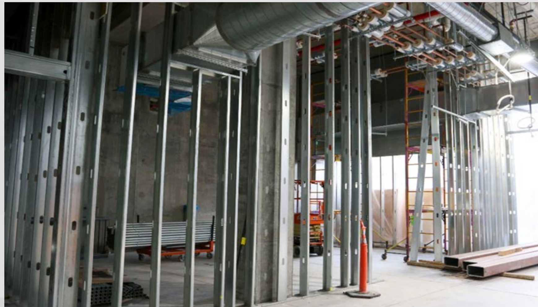
Area G Level 0 Framing
