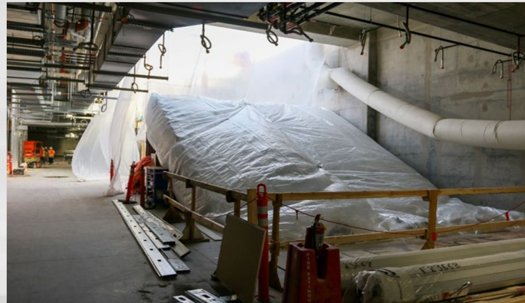
Area G Level 0 Escalator Installation
