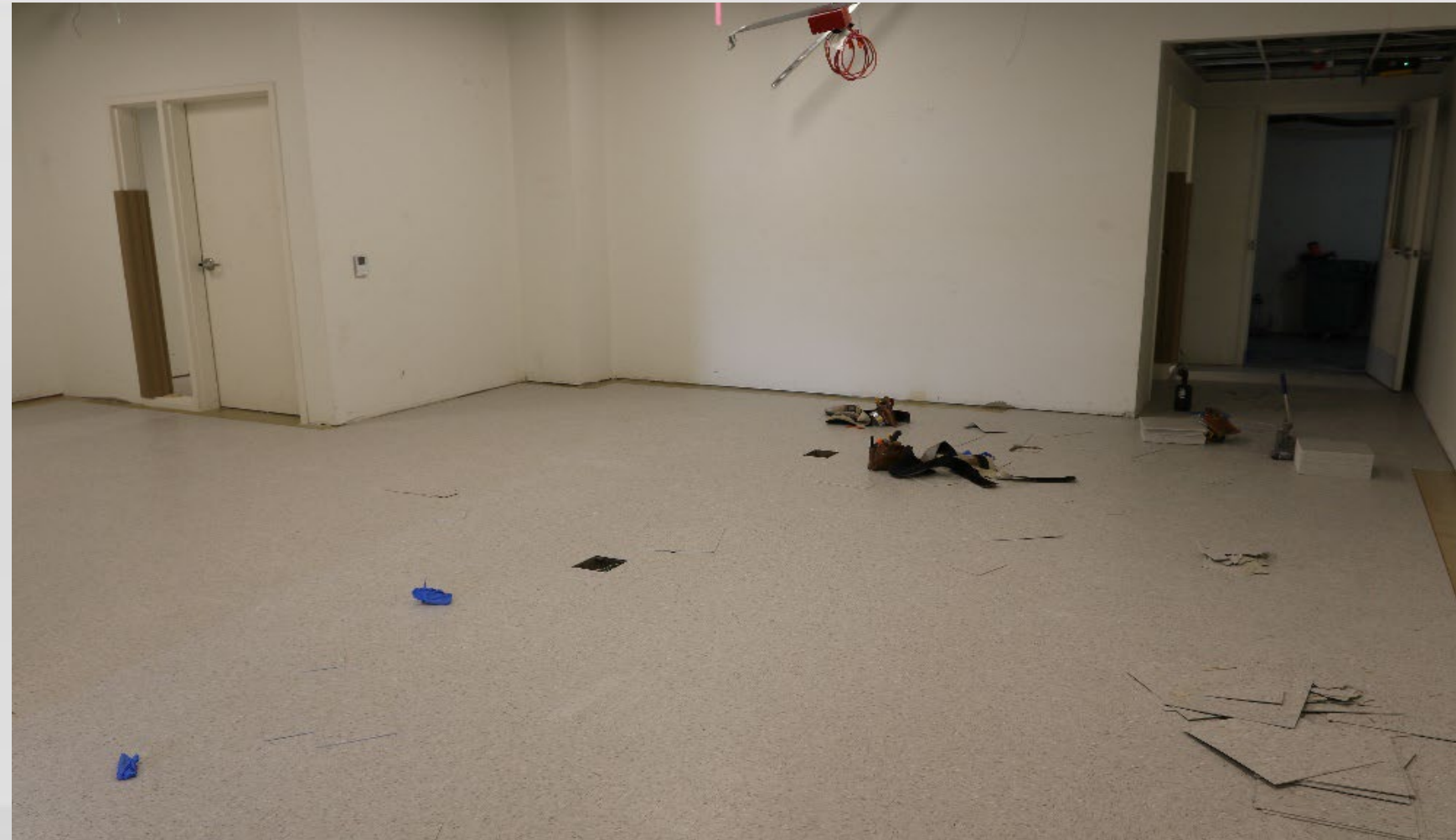
Area C Flooring Installation
