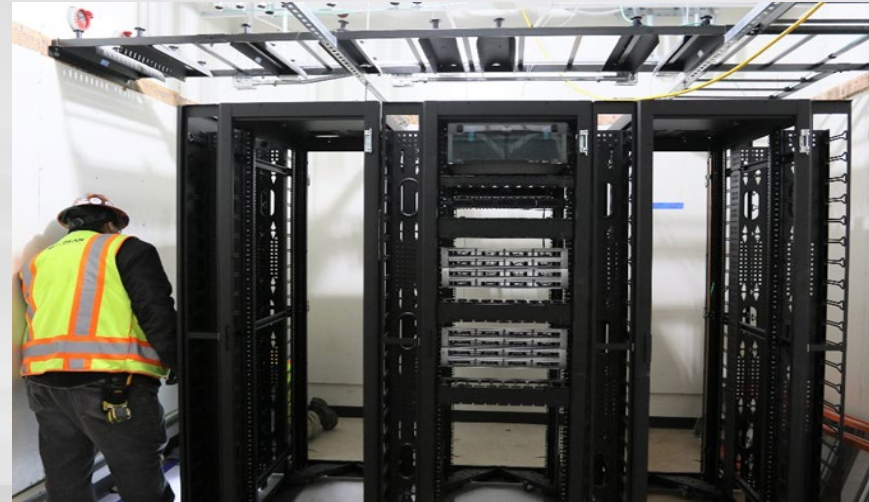
Area F Comm Room Rack Installation
