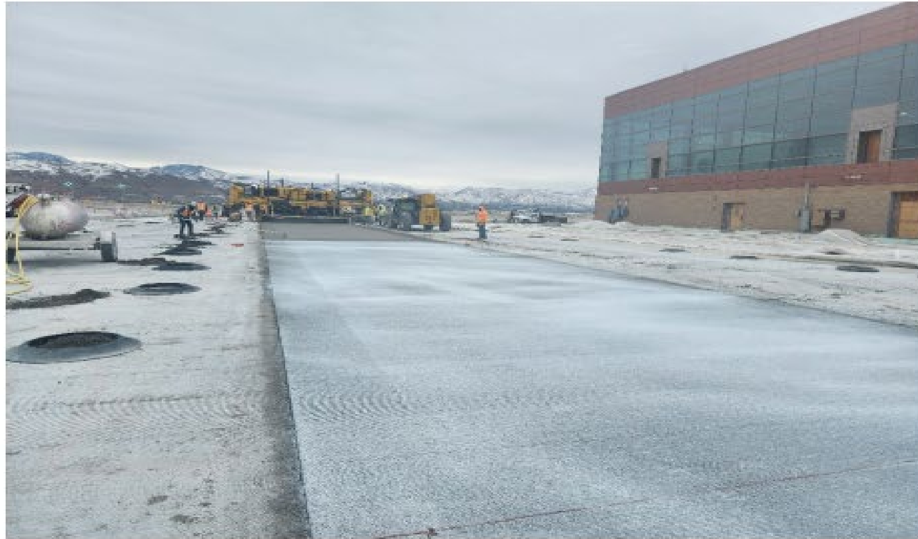
DP11 – North SCE – Placing P-501 Lane AR/183-198
