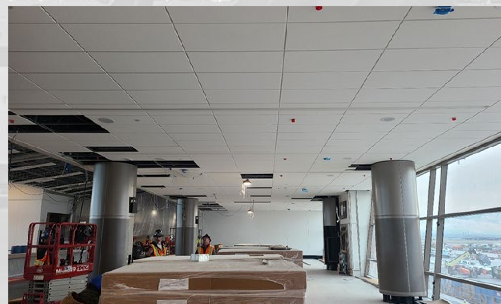
Holdroom Ceiling Installation
