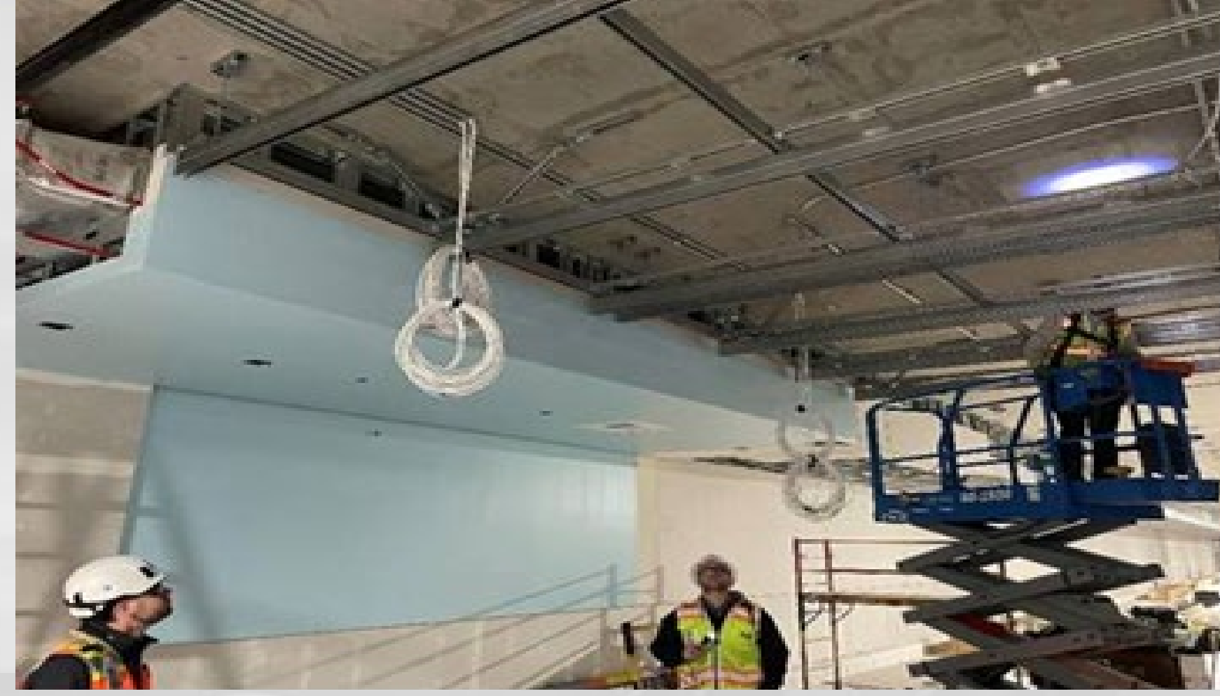
Main Walkway Ceiling Mock-up Installation
