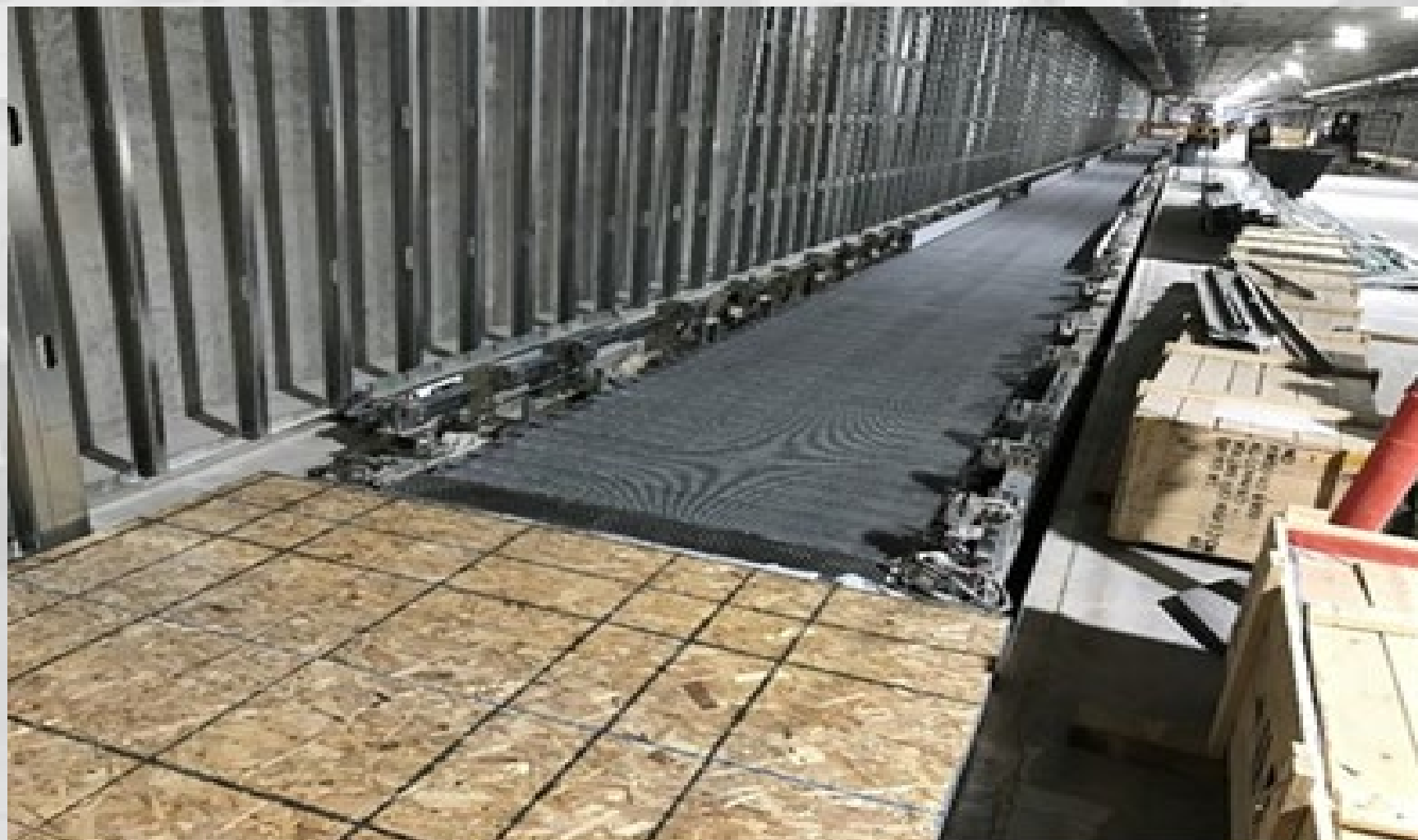
Moving Walk Pallet Installation
