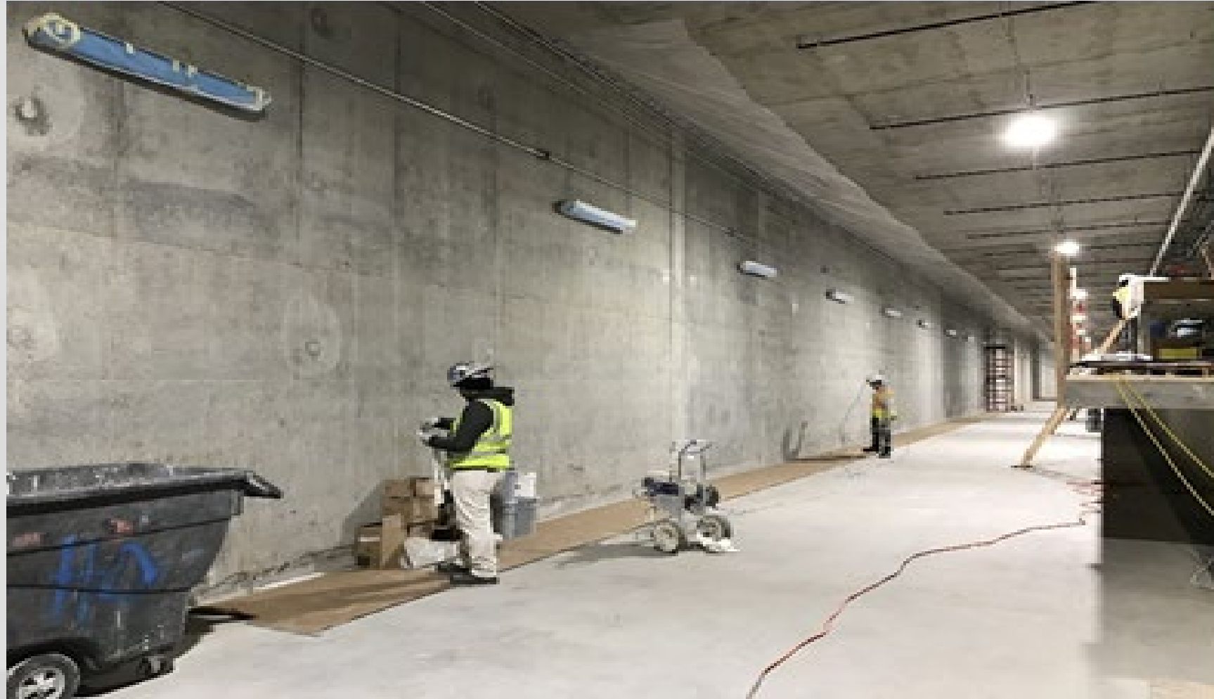
APM Wall Paint Prep
