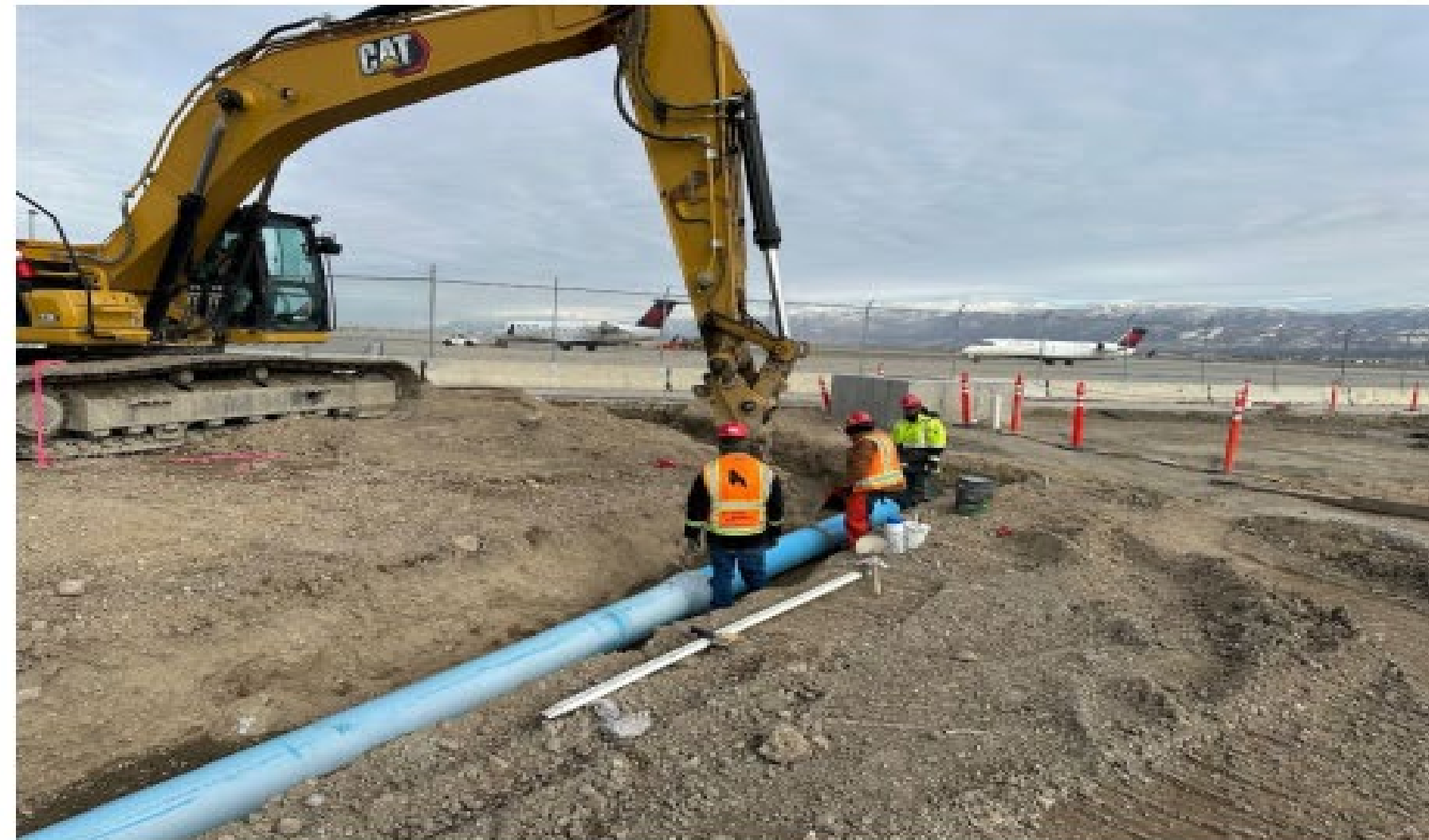
DP11A – NC Phase 4 – Installation of 12" Waterline
