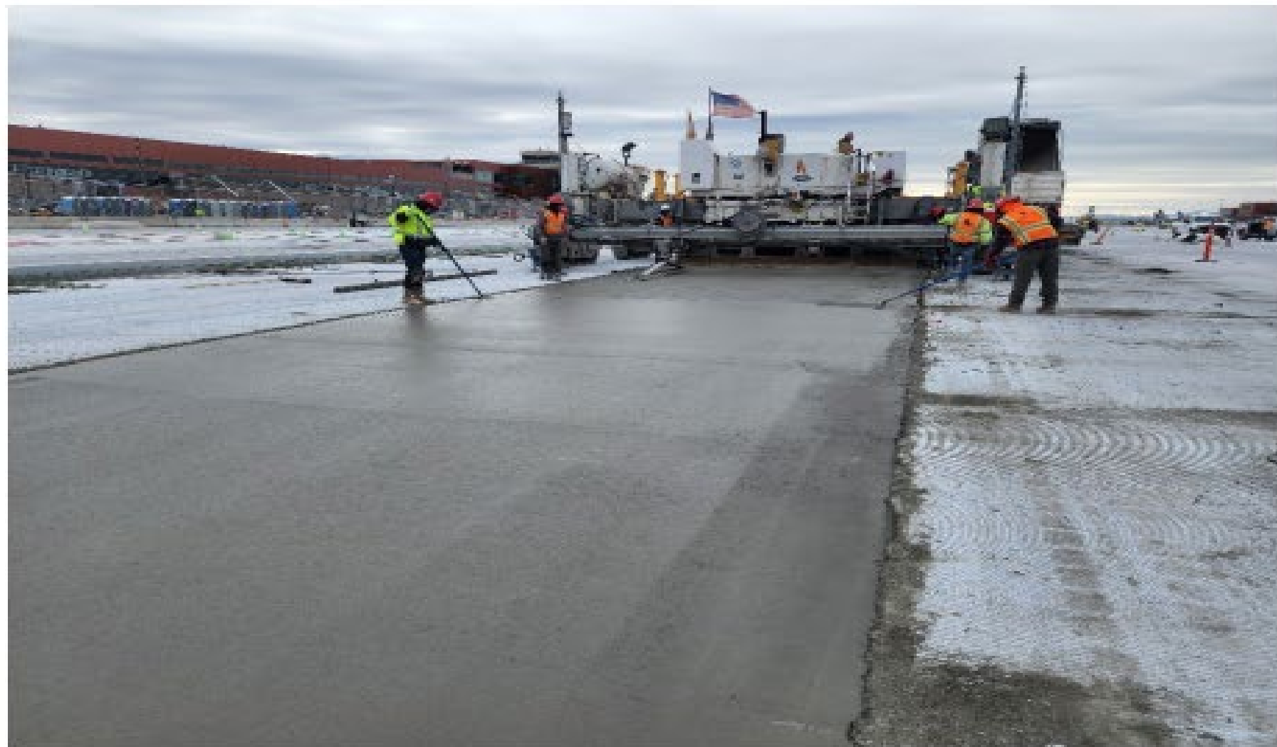
DP11A – Area 2-3 – Placing P-501 Lane AB
