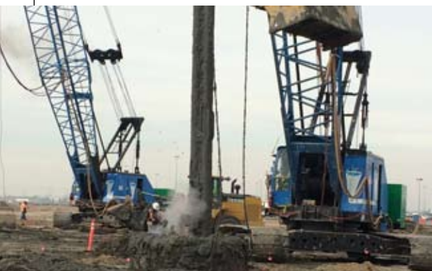
Steel columns are being driven into place.
