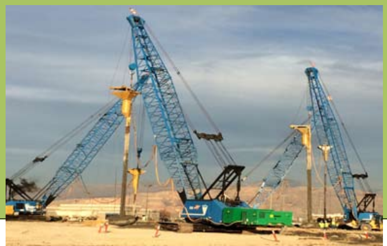
Large cranes are preparing the car rental facility construction site.
